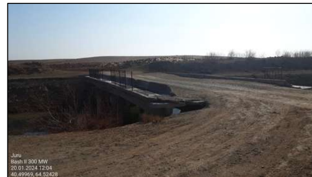
Figure 12-2 Bridges Crossing the Water Channels in the Project Area
