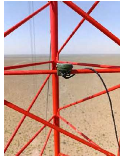
BD02 (North mast - 60 meters)
