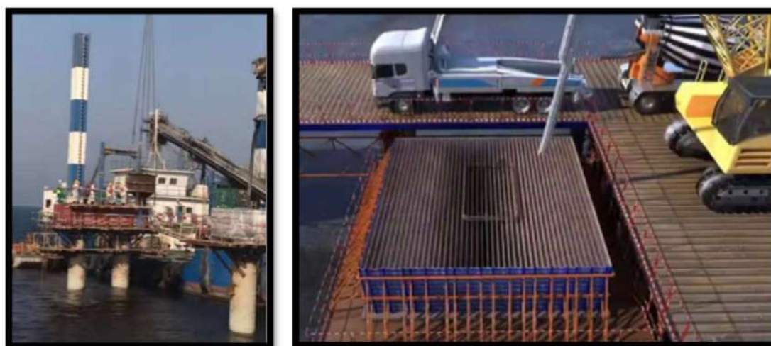
Figure 1.21 Pile Cap Construction
