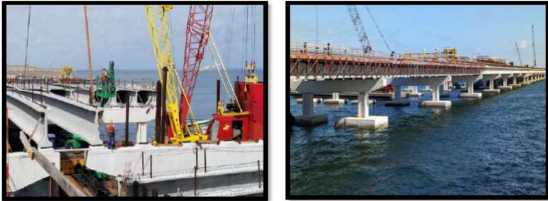
Figure 1.23 Installation of Girders
