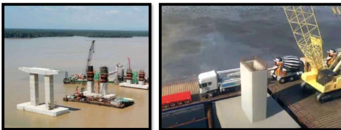
Figure 1.22 Construction of Piers and Pier Head
