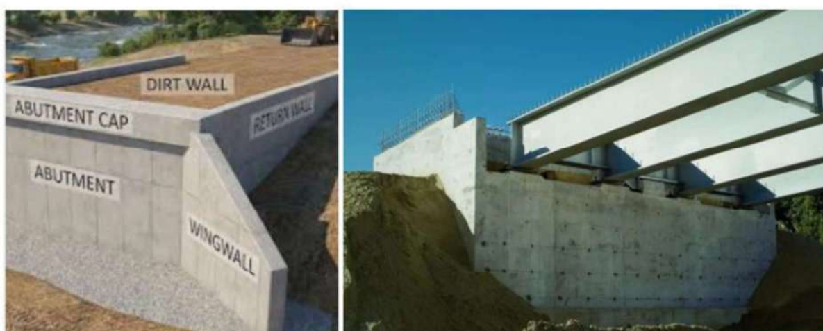
Figure 1.20 Construction of Abutment and Wingwall
