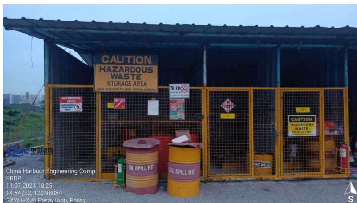
Plate 1-3 Existing Hazardous Waste Storage in the Project Site
