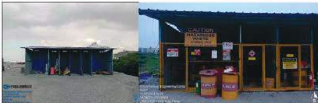
Plate 2-1 Existing Materials Recovery Facility and Hazardous Waste Storage in the Project Site
