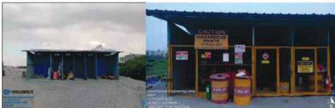
Plate 3-1 Existing Materials Recovery Facility and Hazardous Waste Storage in the Project Site
