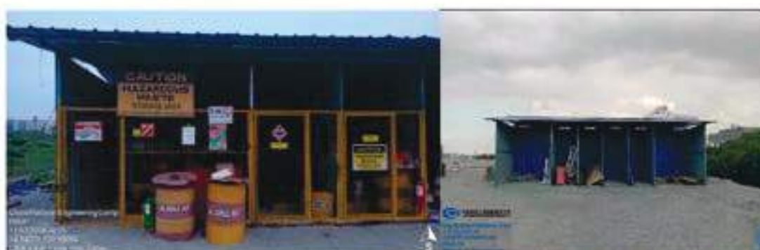
Plate 2-1 Existing Materials Recovery Facility and Hazardous Waste Storage in the Original Island A
