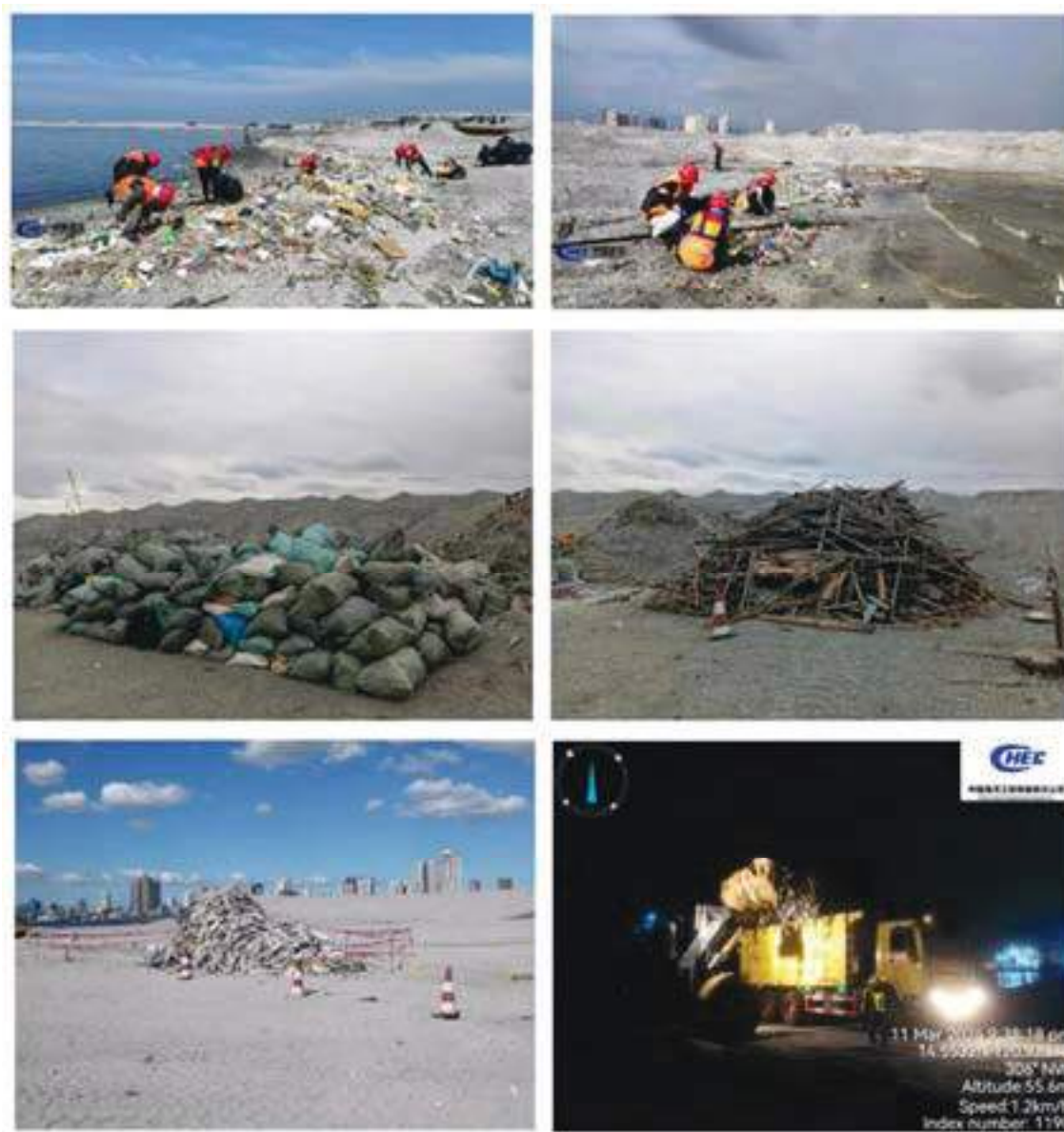
Plate 1-9 Existing Clean-up Activities from the Waste Collected from the Sea and Disposal of Extracted PVD Materials
