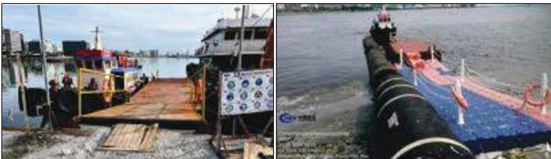
Plate 2-4 Jetty Steel Type (Left) and Jetty Pontoon Type (Right)
