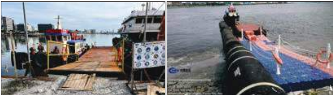
Plate 1-4 Jetty Steel Type (Left) and Jetty Pontoon Type (Right)
