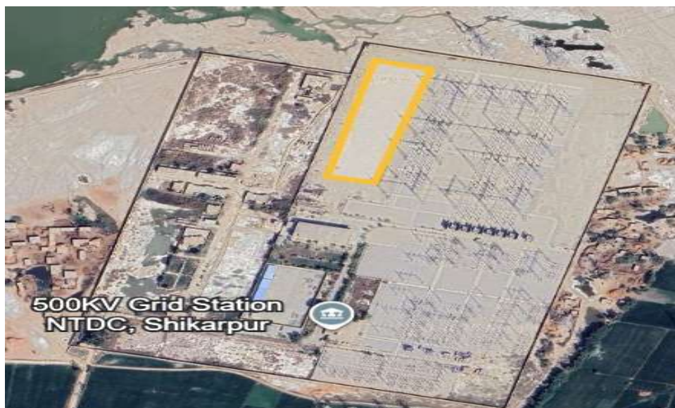
Satellite Image of 220kV Shikarpur GS
