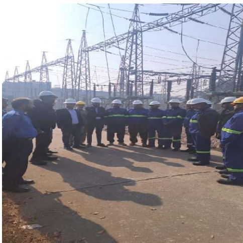
Consultation at 220kV Ravi Road GS
