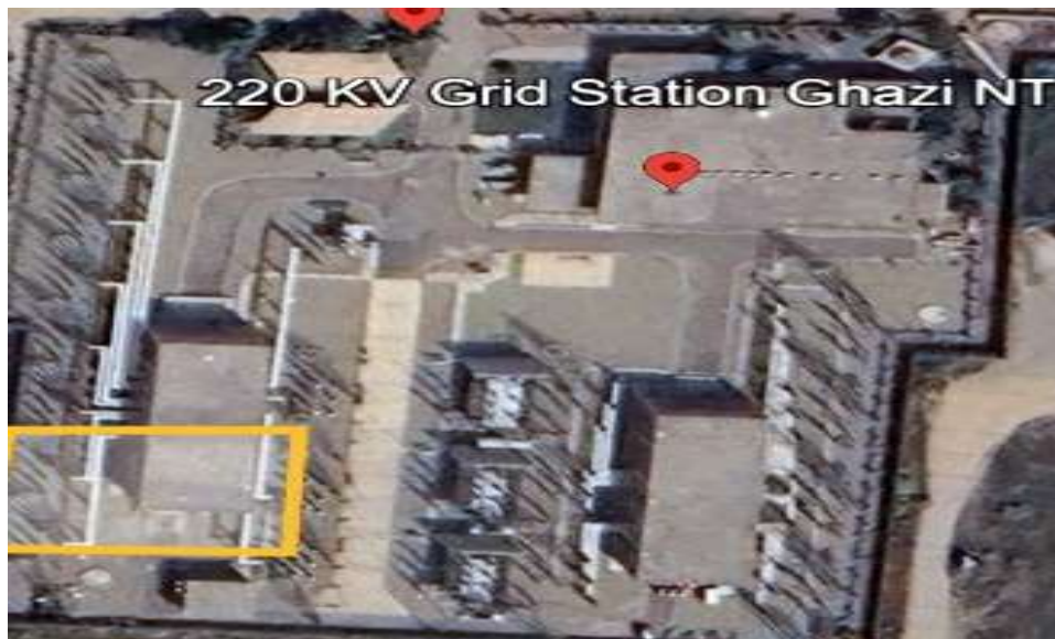
Satellite Image of 220kV GS Ghazi Road
