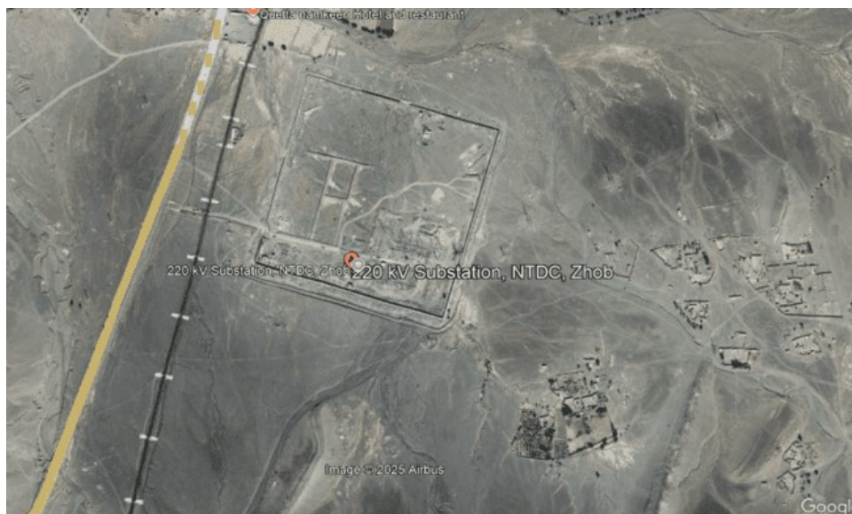
Satellite Image of 220kV GS Zhob
