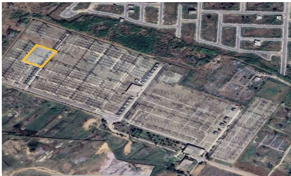
Satellite Image of 500kV GS Rawat
