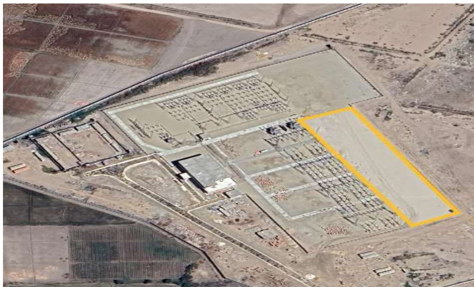
Satellite Image of 220kV GS Mirpur Khas
