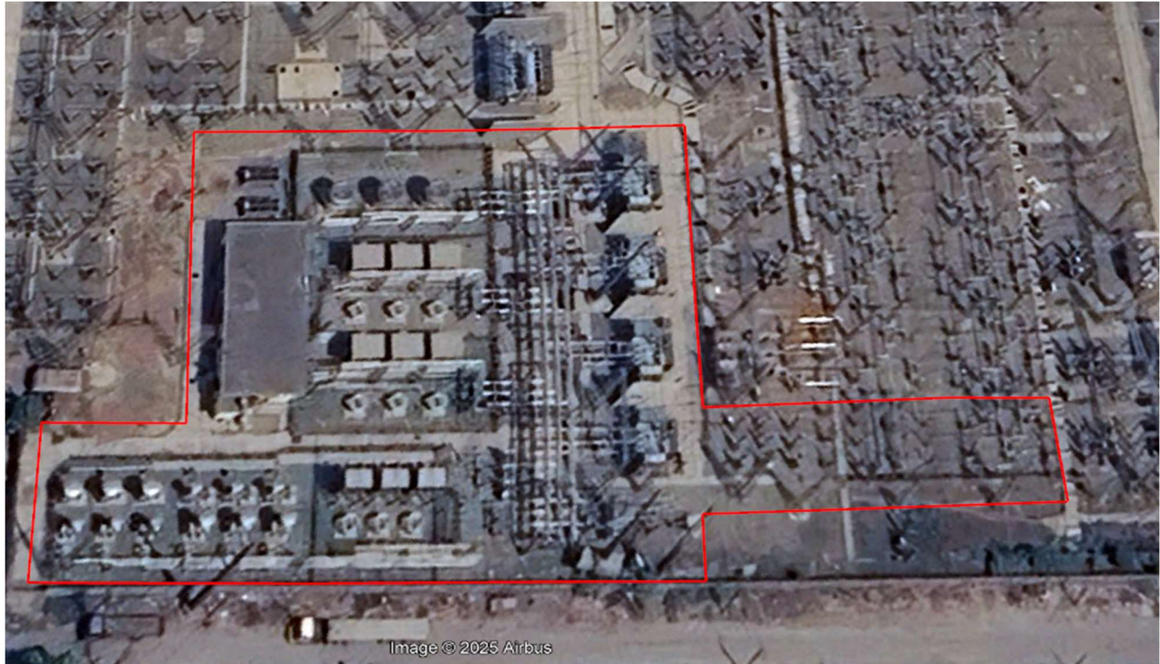
Figure 2-2 Satellite Imagery of SVC in NKLP
