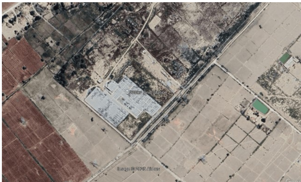
Satellite Image of 220kV GS Dera Murad Jamali
