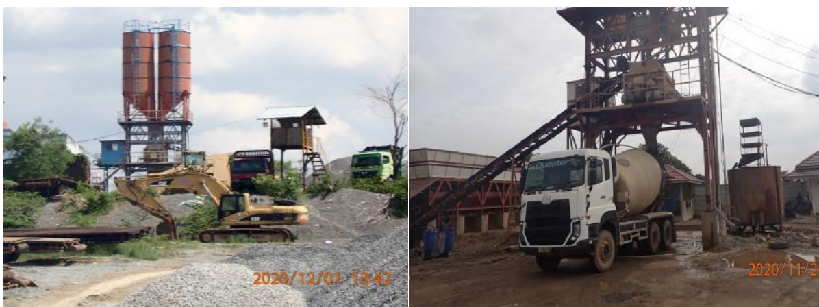
Figure 16 Concrete Batching Plants
