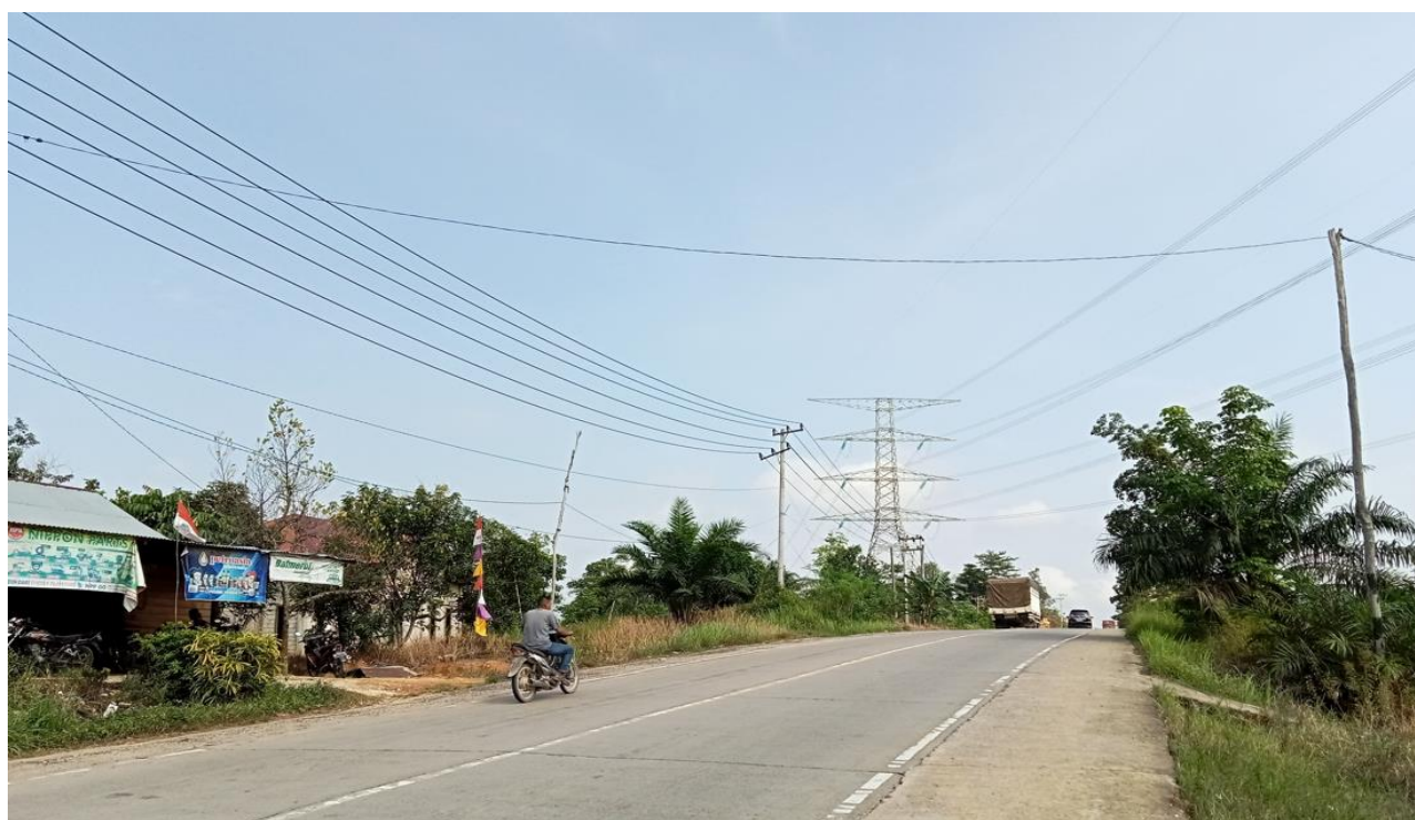
Figure 27 Typical Condition of Trans Sumatera Road
