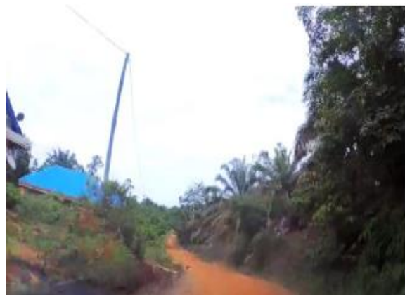
Part of unpaved access road from Trans Sumatera National Road to ~STA 50+000
