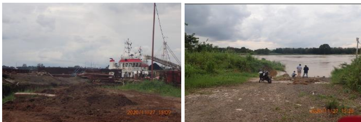
Figure 17 Typical Jetties at Batanghari River
