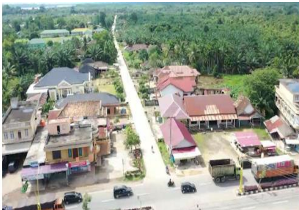
Access road of asphalt pavement from Trans Sumatera National Road to ~STA 17+000
