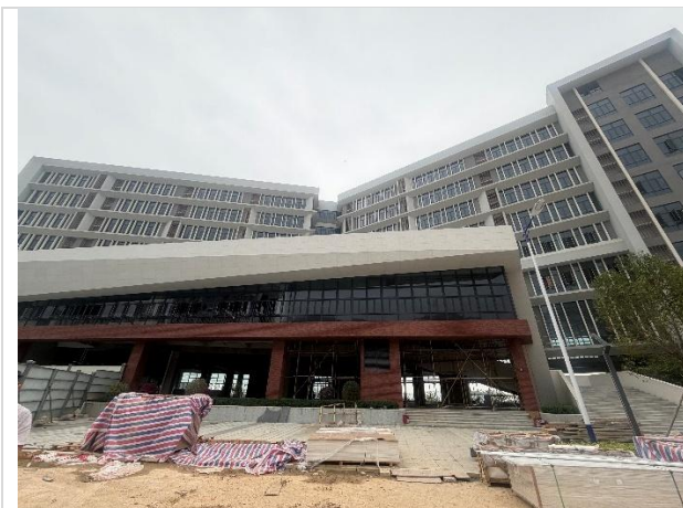
Photo 1: Completed building in the construction site
