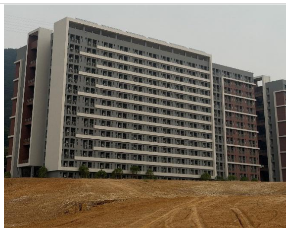
Photo 2: Completed building in the construction site
