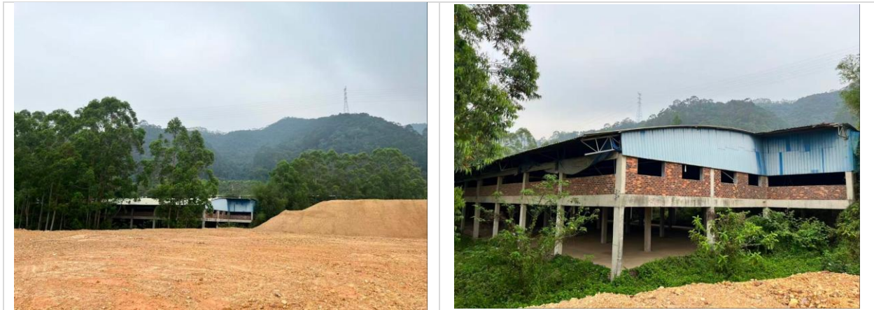
Figure 3-1 Current Status of the Unrelocated Pig Farm within the Project Area
