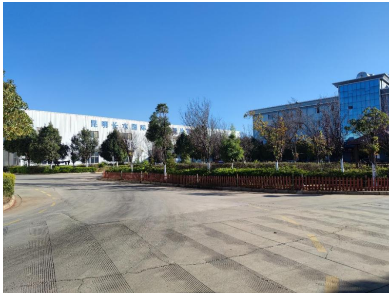
Fig. 4 Overview of domestic waste treatment station
