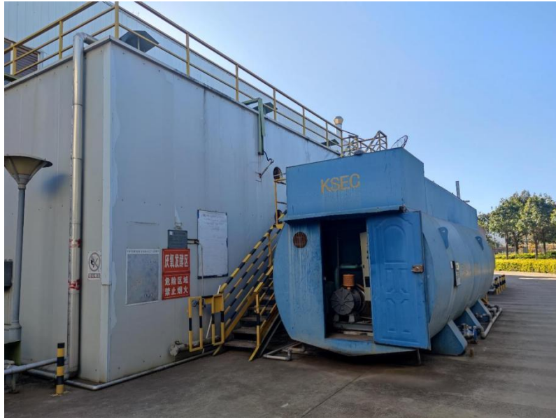
Fig. 7 Domestic waste leachate treatment device
