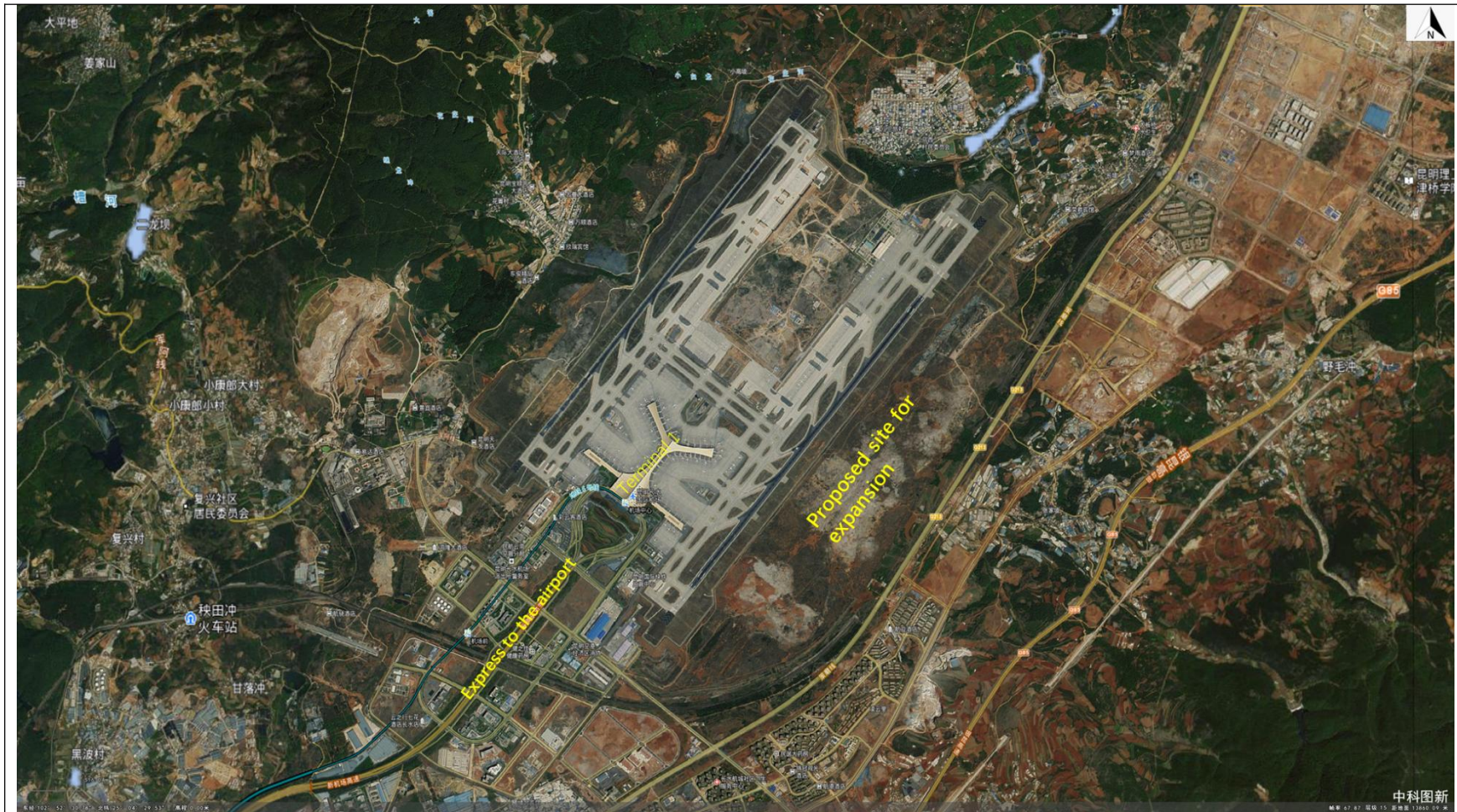
Fig. 1 Satellite image of the site and vicinity
