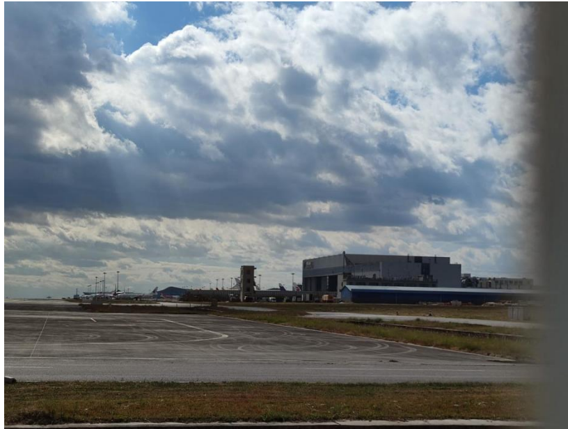
Fig. 13 China Eastern Airlines Maintenance Center (no access inside)
