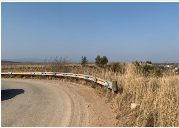
Site of East Runway #2
