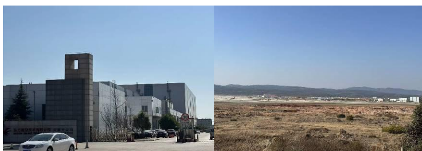
Figure B-1 Current Situation of the aircraft maintenance station and Available Unused Land
