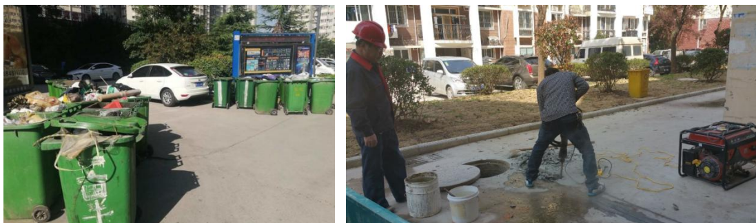
Figure 14-6 Community Waste Disposal and Water Pipe Maintenance
