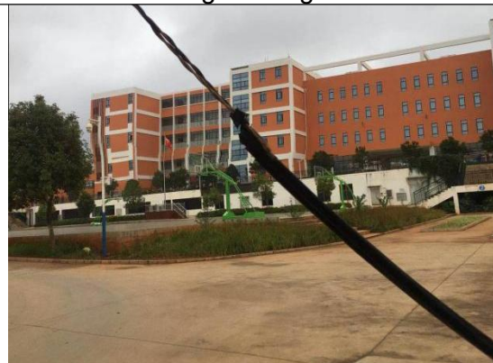
Kunming Airport No.1 Primary School (sound insulation measures have been installed)
