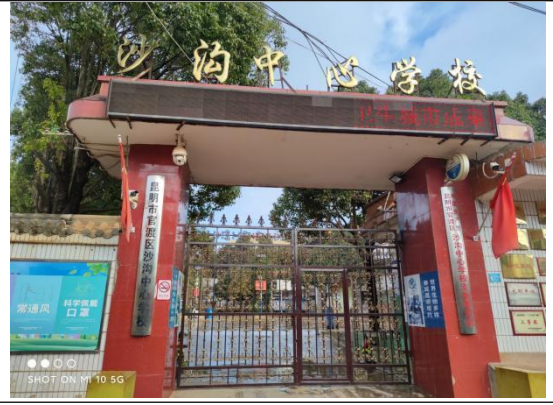
Shagou Central School (sound insulation measures have been taken)
