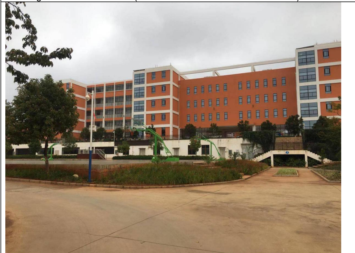
Kunming Airport No.1 Primary School (with sound insulation windows installed)
