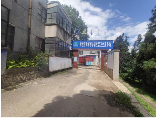
Xiaoshao Township Hospital (sound insulation measures)
