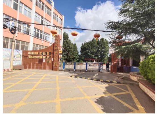
Kunming Guanghua School (sound insulation measures)
