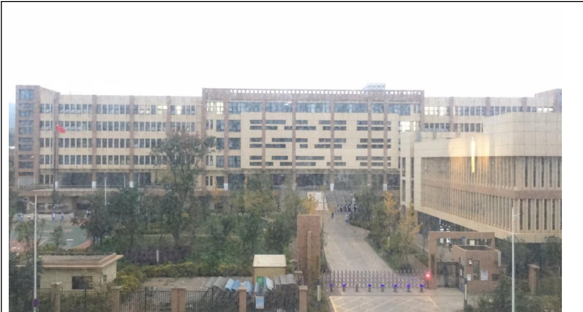
Kunming No. 17 Middle School (with sound insulation windows installed)
