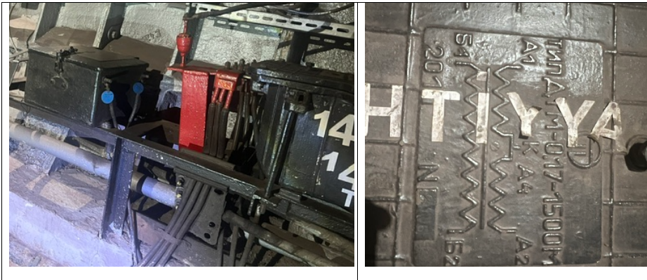
Figure 2: Drossel-Transformer DTM-0.17-1500
