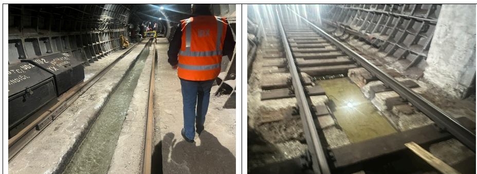
Figure 6: Drainage in Baku Metro Tunnels
