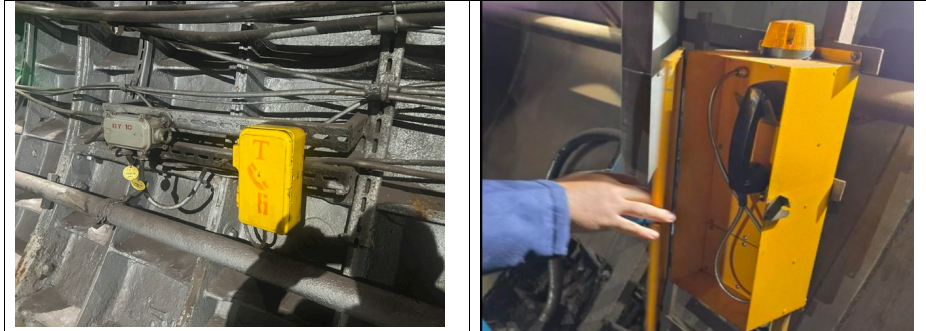
Figure 5: Tunnel Telephones
