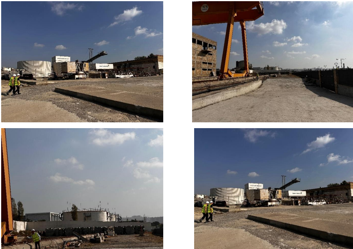
Figure 5-4 Y-15 Ongoing Construction Activities and Vicinity
