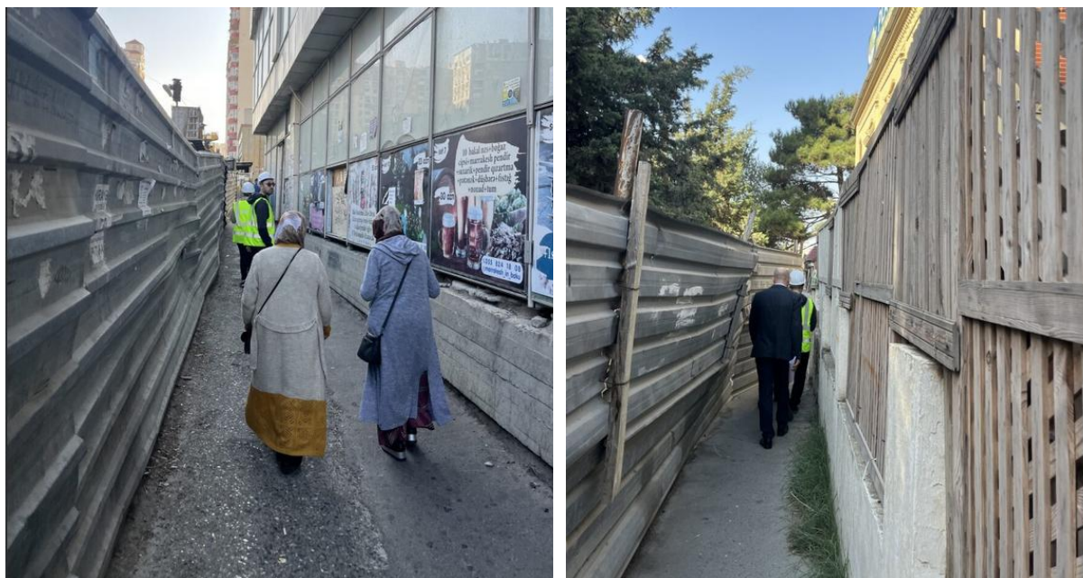
Figure 5-10 Y-16 – Temporary Impacts of Construction, Narrowed Roads
