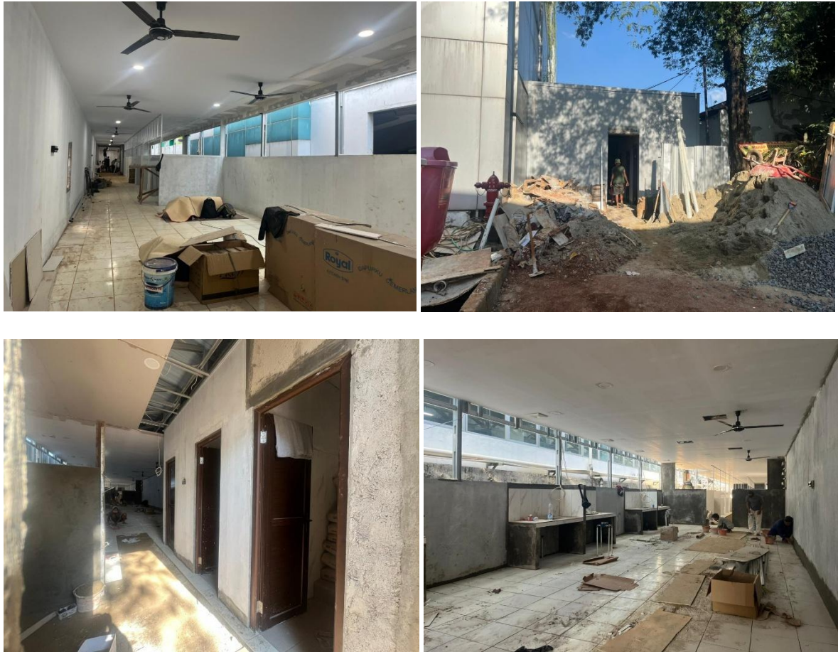
Figure 12. Canteen Construction Process
