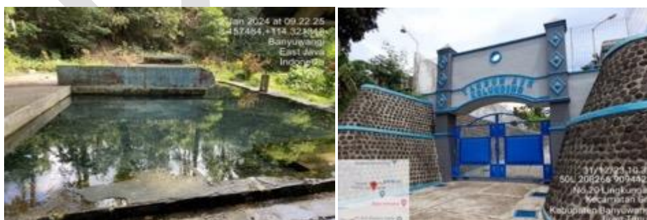
Figure 4-110 Clean water source facilities in Kelir Village (left) and clean water facilities in Giri Village (right)
