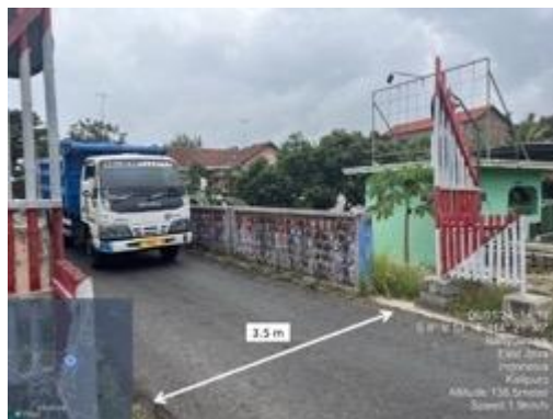
(c) Bridge condition at Joyoboyo Road
