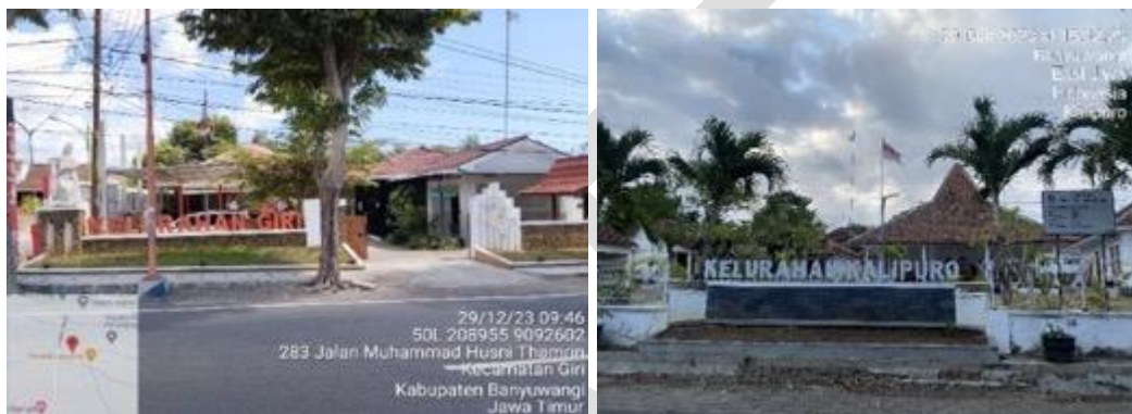
Figure 4-106 Village Government Offices in Giri Village (left) and Kalipuro Village (right)
