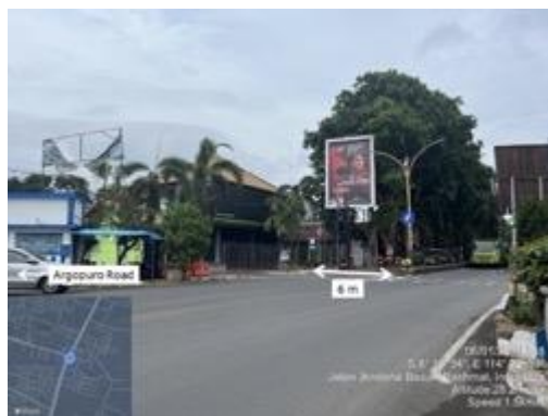
(a) Raya Banyuwangi – Situbondo Road condition (TR2)
