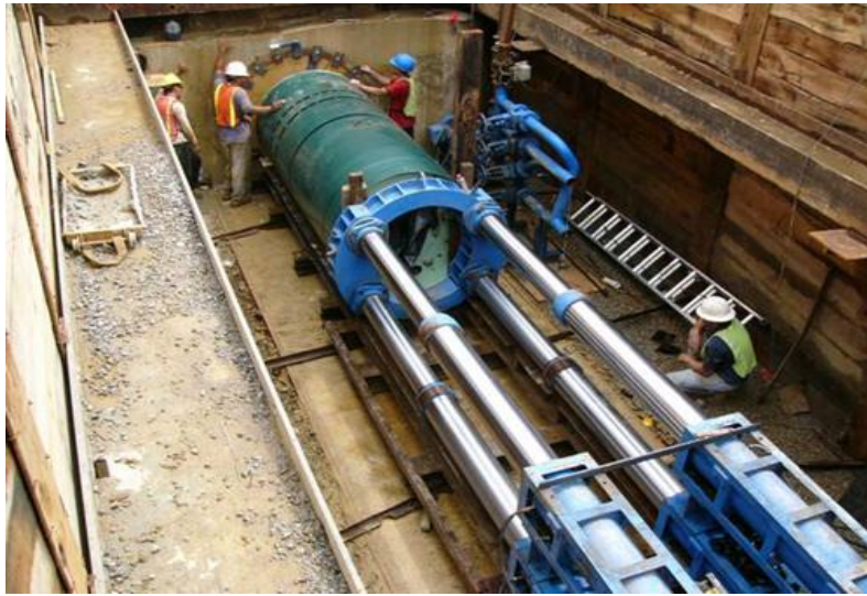
Figure 3-9: Typical Jacking Frame
