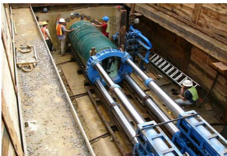
Figure 3-9: Typical Jacking Frame
