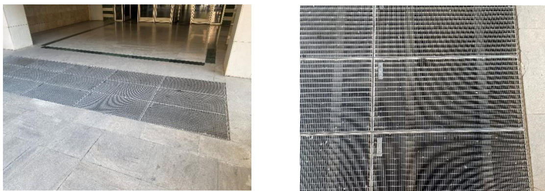
Figure 1: Drains at Station Entrances
