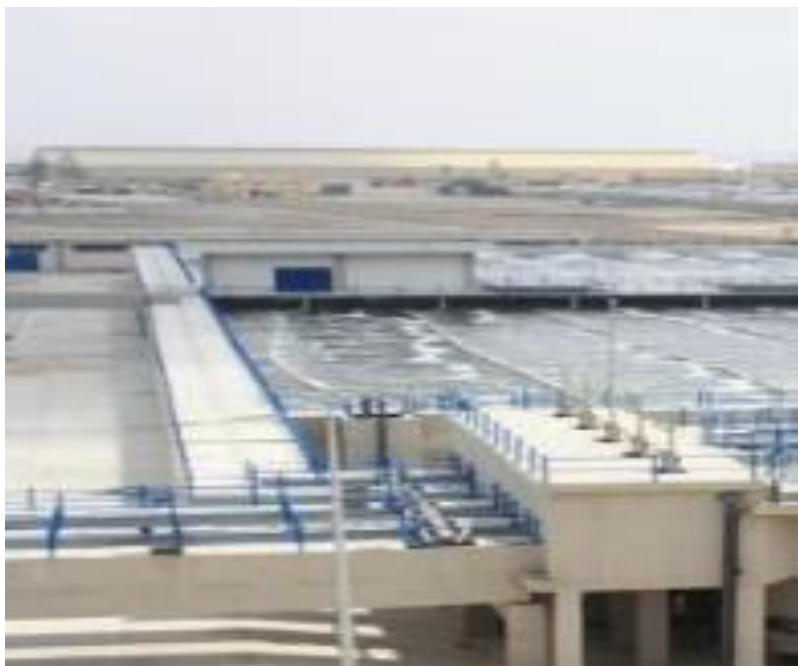
Figure 18: Example of distribution unit
