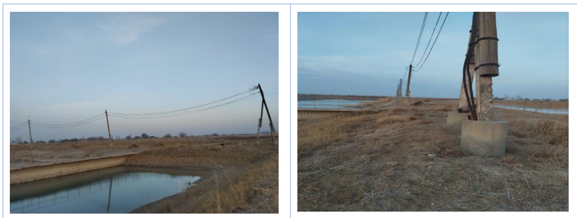
Figure 5: The water intake "Aydin-Zhol" located in Takhiatash district
