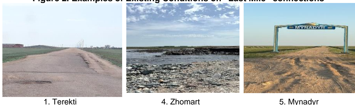
Figure 2. Examples of Existing Conditions on “Last Mile” connections
