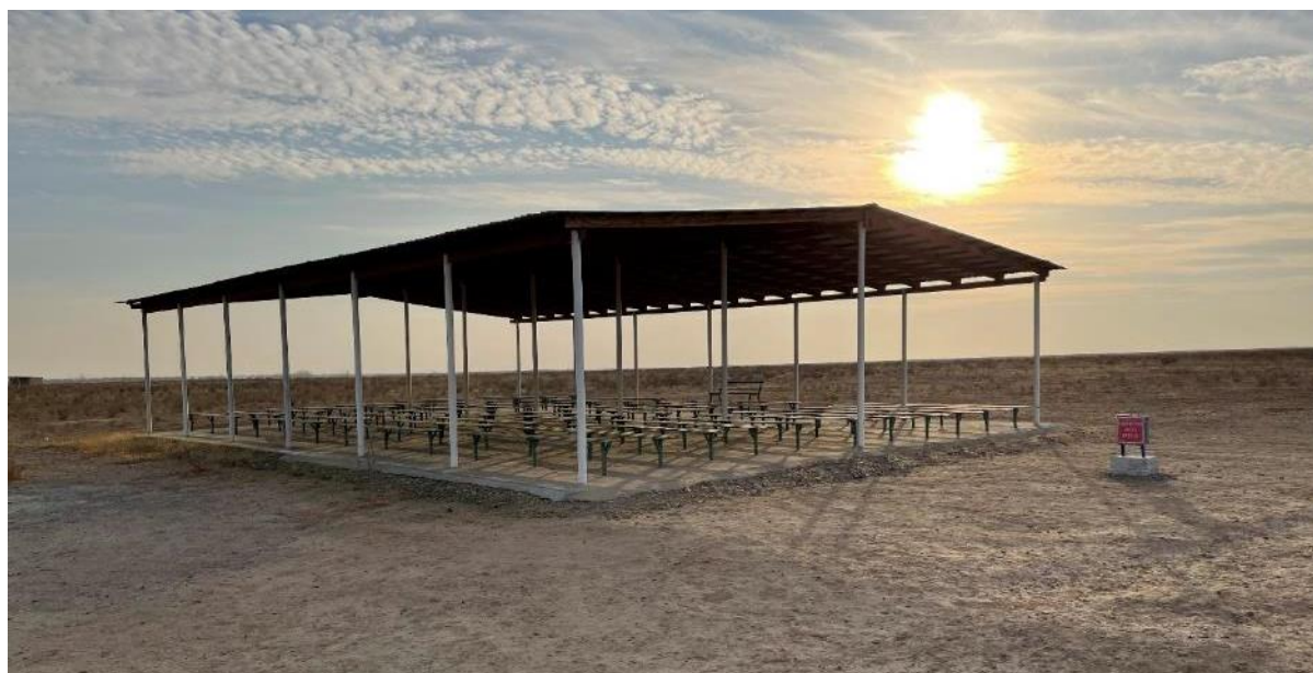
Figure 6-53. Prayer area attached the cemetery in the middle of the project site
