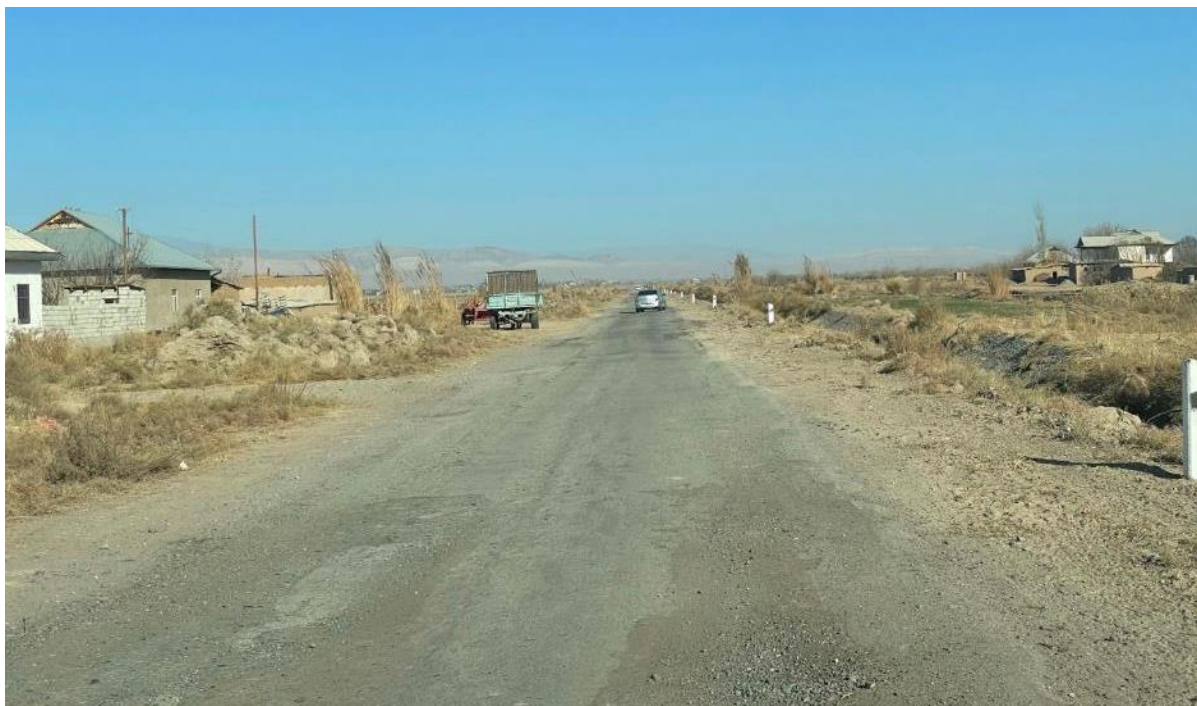
Figure 6-62. Minor road on the approach to the site
