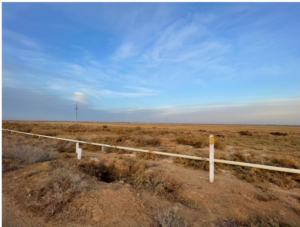
Figure 6-55. General character of the transmission line route (Dec 2021)
