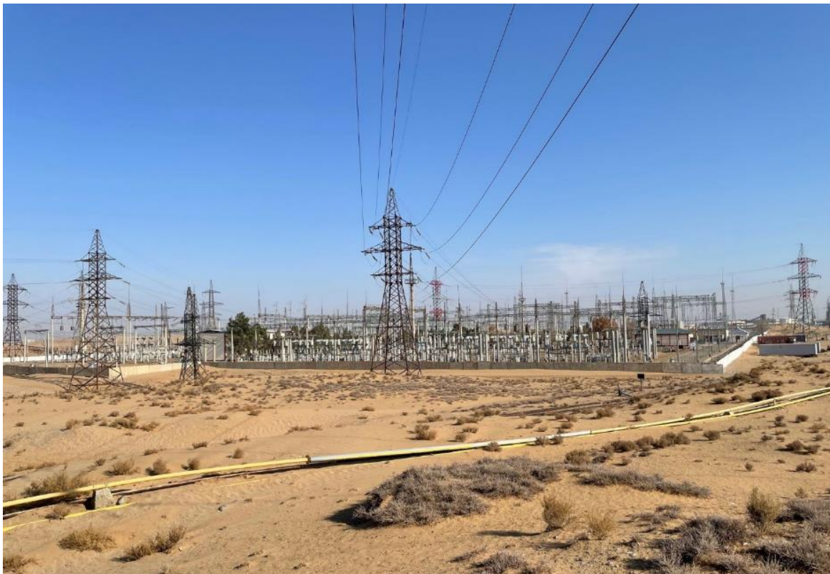
Figure 2-18. Connection point at the Surkhan substation
