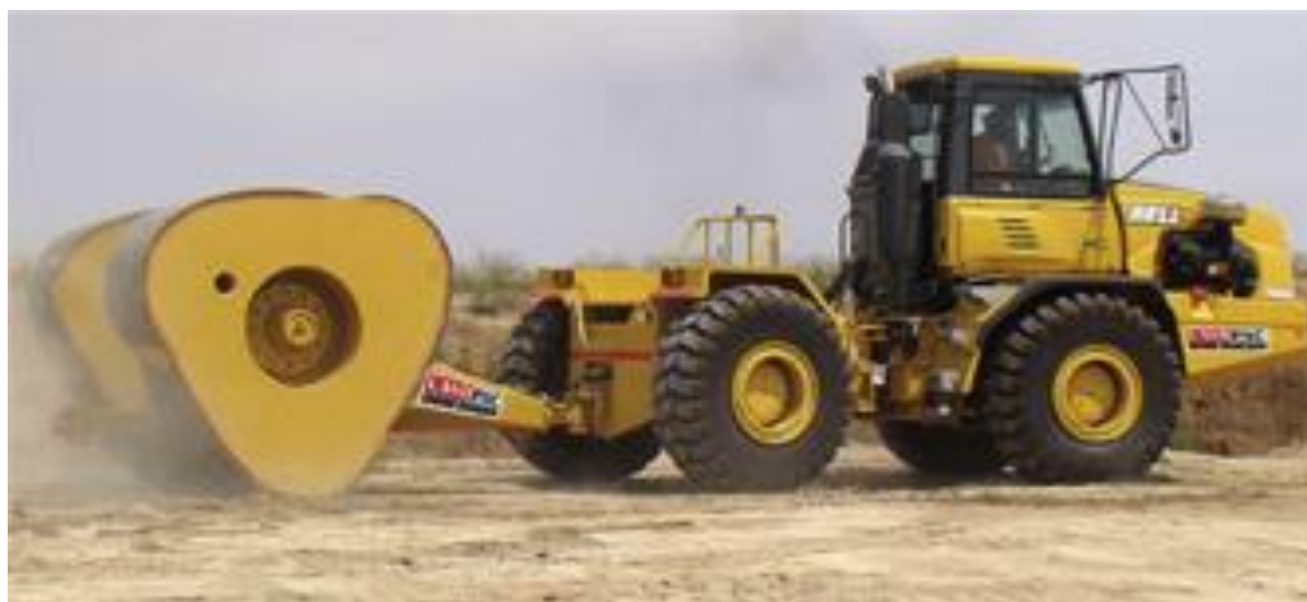
Figure 2-21. Rolling dynamic compaction (RDC)
