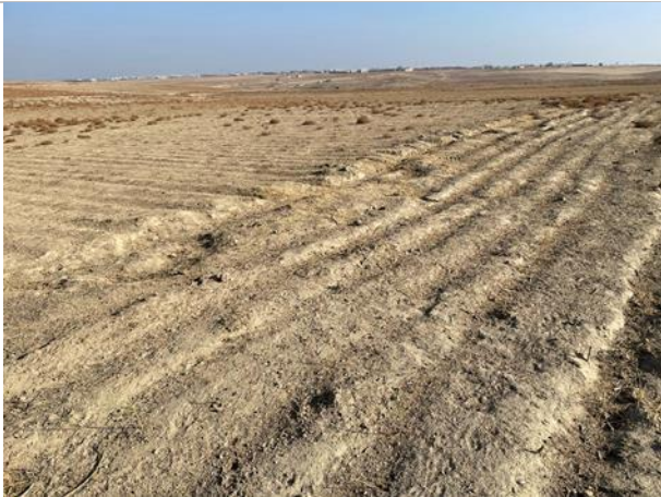
Figure 6-3 Land preparations by leaseholder 4 in the Solar PV Area
