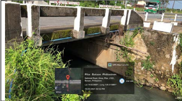
K0133+350 (Catmon Bridge)
