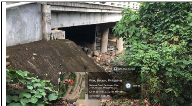
K0137+013 (Pantingan Bridge)
