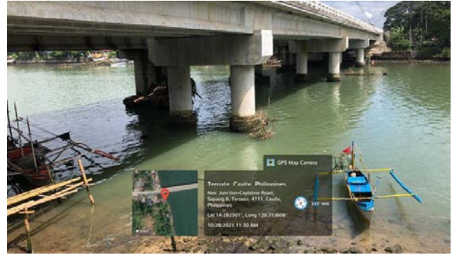
K0056+157 (Maragondon Bridge)
