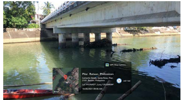
K0132+450 (Orion Bridge)
