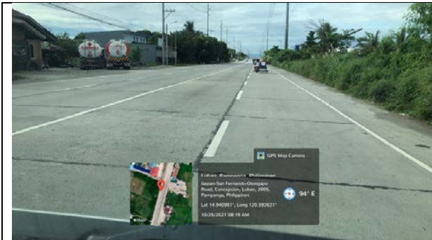
K0086+900 (Santa Cruz Bridge)
