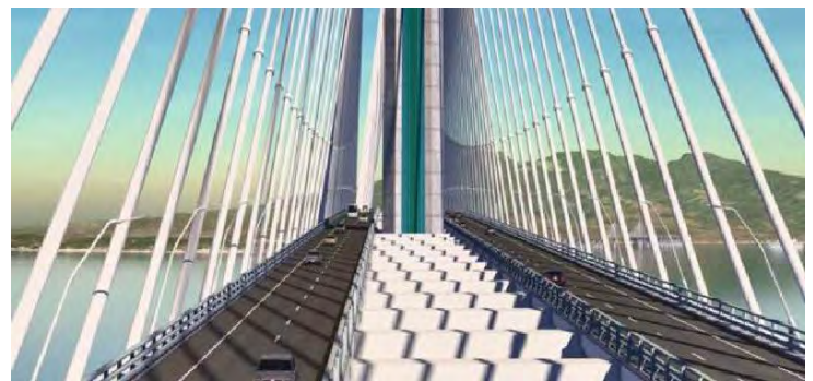
Exhibit 3-18 South Navigation Channel Bridge Deck showing Steel Box Girders with Cross-struts
