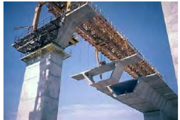
Exhibit 3-17 Launching Gantry Installing Precast Concrete Box Girder Segments
