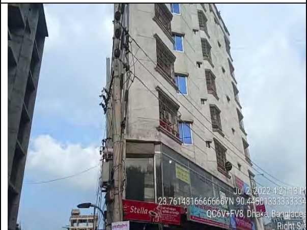
Beside Rampura Police Box Main Road, Dhaka (C/S -203 Chainage 10+100km)
