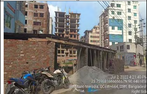
Alif Stand Meradia, Dhaka (Beside C/S -198 to -199 Chainage 09+850km to 09+900km)
