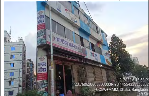
Meradia Bazar Road (C/S -201 Chainage 10+000km)
