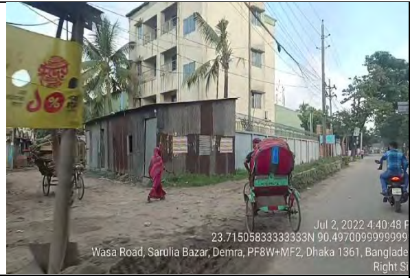
Wasa Road, Sarulia Bazar, Demra (Beside C/S -46 to -47 Chainage 02+250km to 02+300km)
