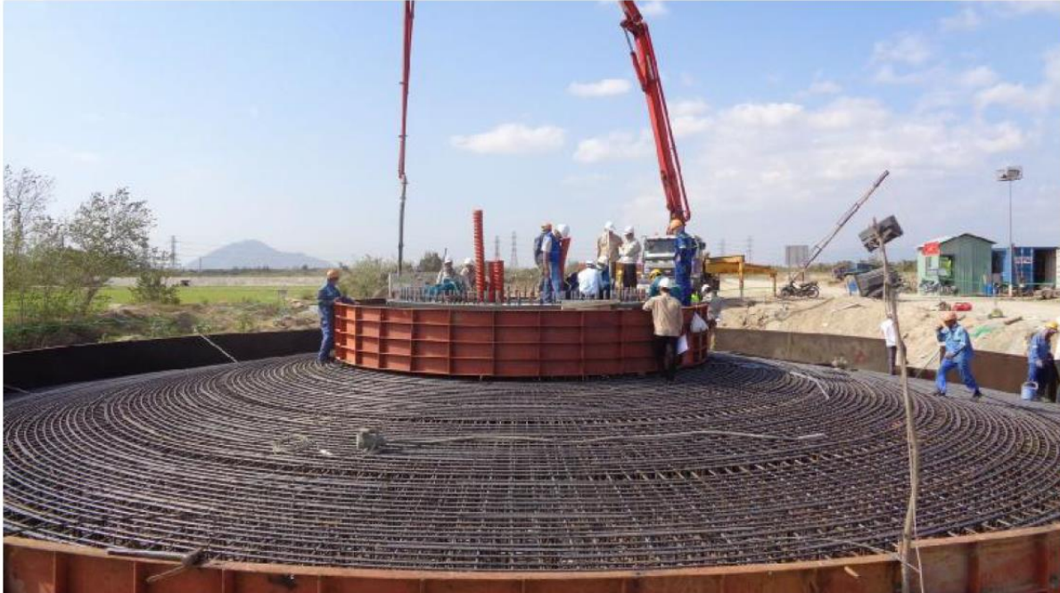
Figure 2.6 Construction of the Wind Turbine Foundation
