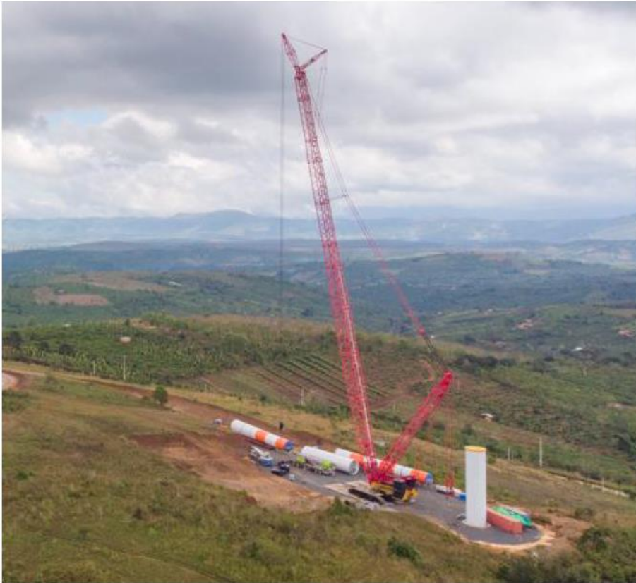
Figure 2.7 Installation of the Wind Turbines
