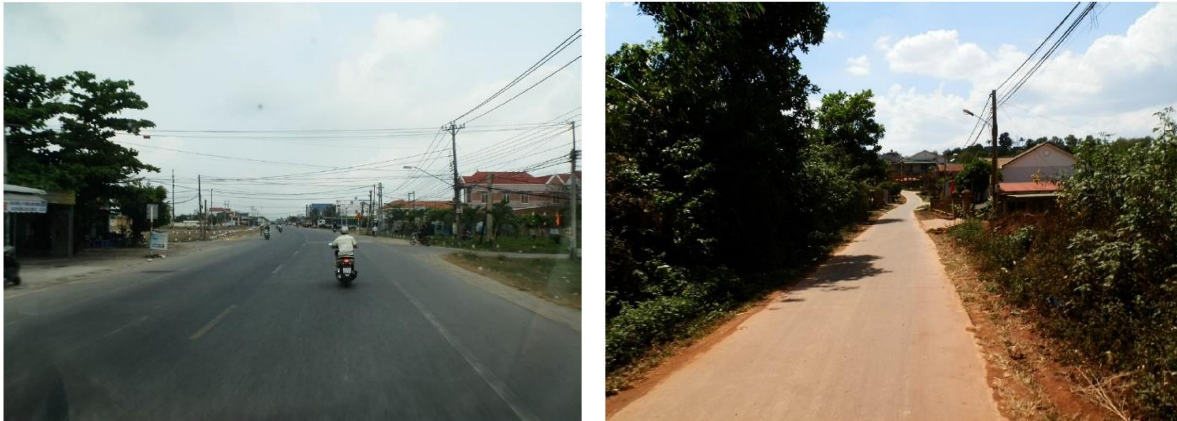
National Highway No.14
