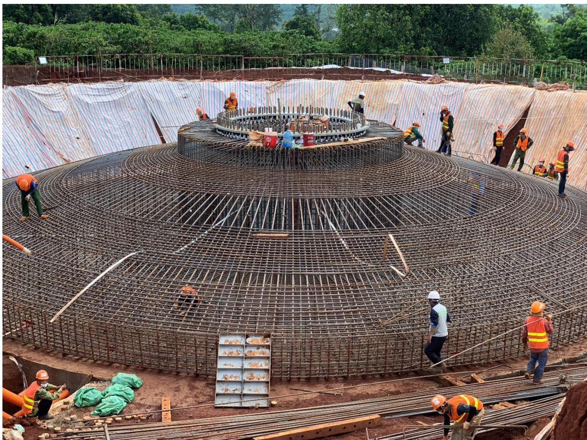
Figure 2.15 Turbine Foundation
