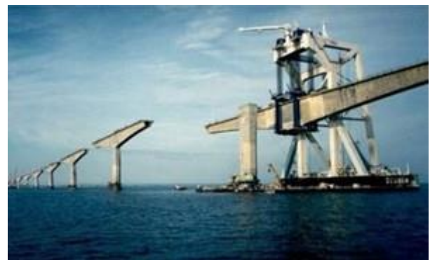
Exhibit 3-15 Full Span Heavy Lift
