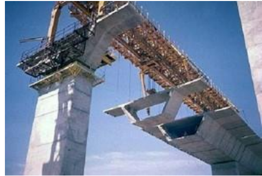
Exhibit 3-16 Launching Gantry Installing Precast Concrete Box Girder Segments
