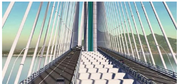
Exhibit 3-17 South Navigation Channel Bridge Deck showing Steel Box Girders with Cross-struts
