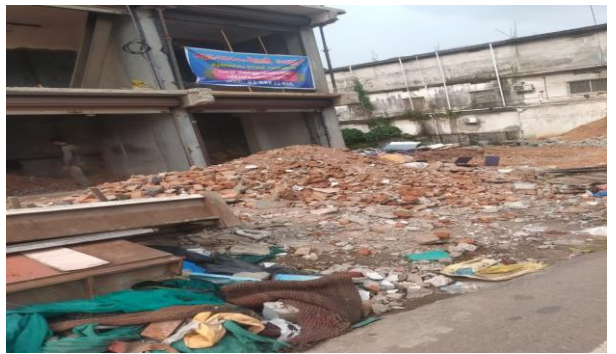
On going demolition work at Vazhakkala
