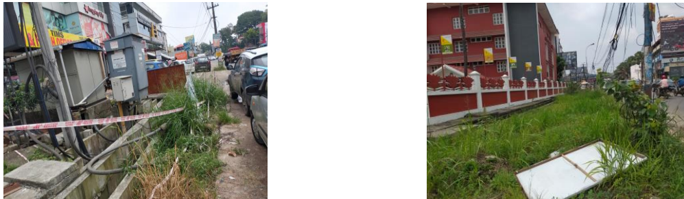
Figure 4.18 Utility Shifting Work is in Progress
