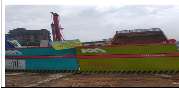
Ongoing piling work at Cochin SEZ station LHS
