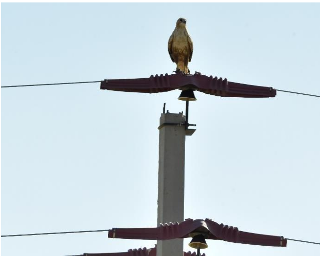
Isolate device for power cap of pillar
