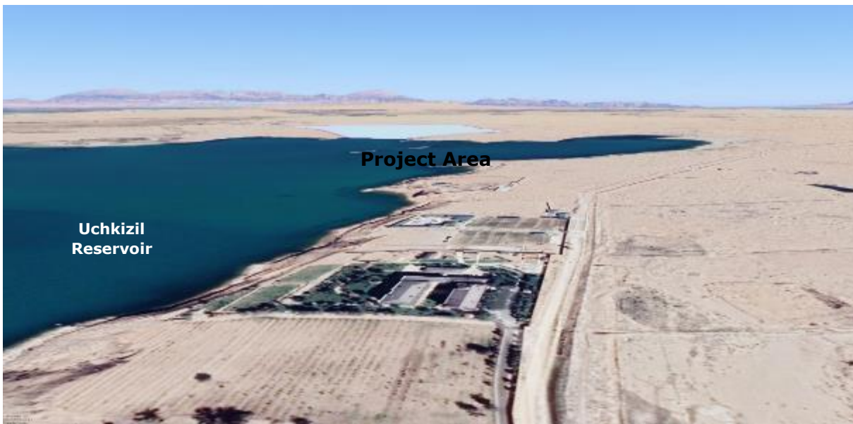
Figure 176: View of the Project Area from the South Direction
