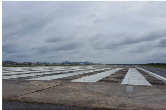
Airsides area at runway no.1 (current)
