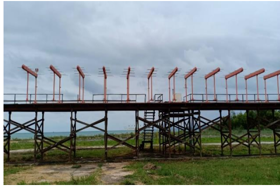
Air navigation aids at the end of the runway no.1 (36L)
