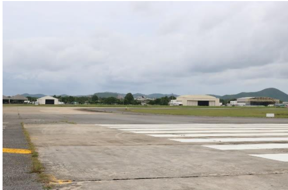
Navy aircraft hangar, on the west side of the runway no.1
