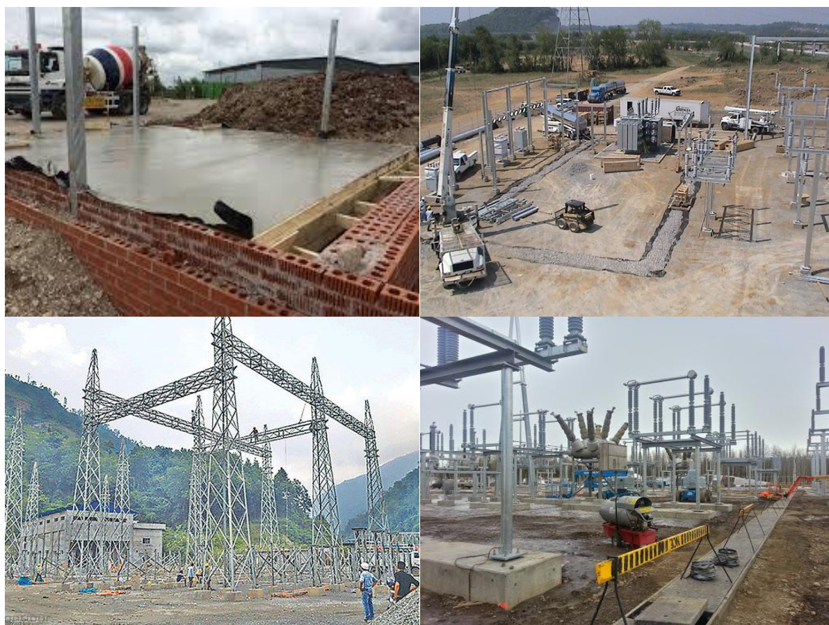
Figure 4-7: Sample Photographs of Construction of Substations
