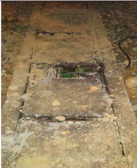
Broken slabs in yard causing health and safety hazard to workers
