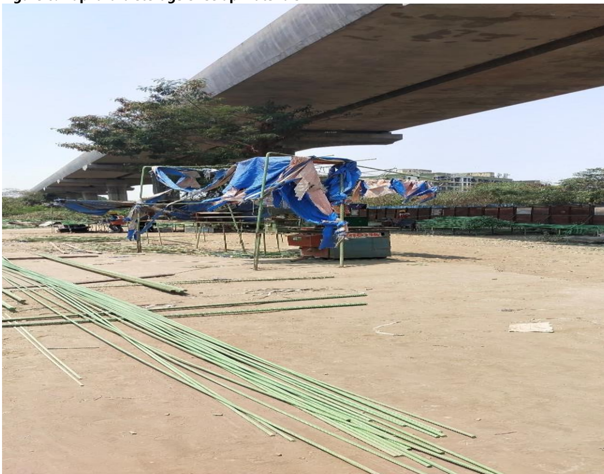
Figure 7: Poorly constructed and fully torn shade for workers
