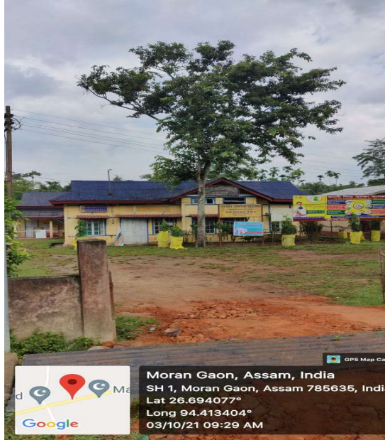
Figure 4-43: Health Centre at Ch. 0.100 km
