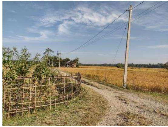
Bypass Section Ch. 15+300
