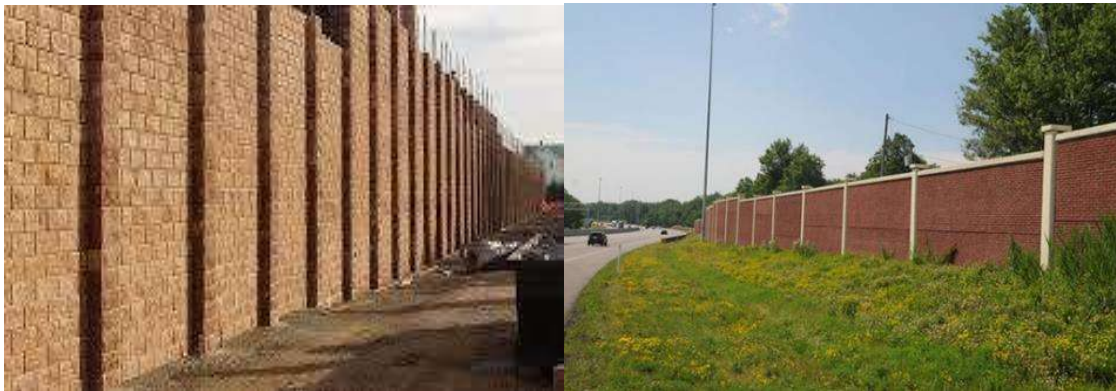
Figure 5.6: Representative photos of Noise Barriers (Bricks type)
