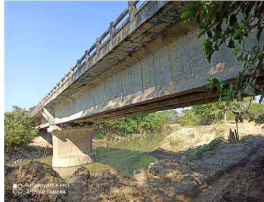
Kaldia River (Ch. 10+400)
