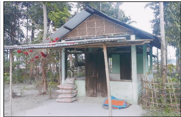
Exhibit-2: Semi-Permanent Structure
