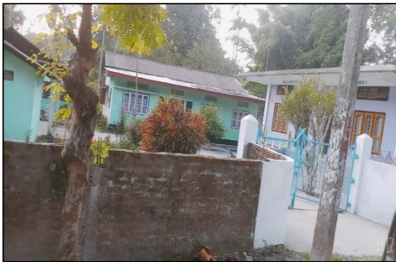
Exhibit-1: Permanent Structure
