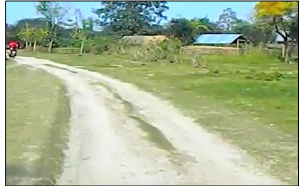
Exhibit-2: Earthen Road
