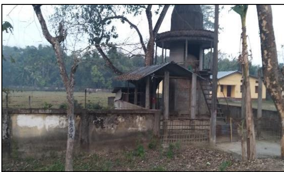
Under construction Temple along the project
