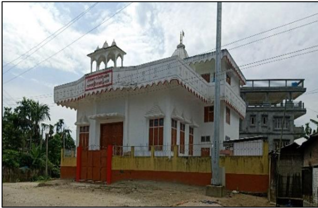
Exhibit-1: Temple Boundary Wall along the
