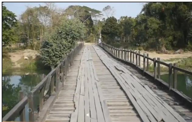
Exhibit-1: Roha Bridge
