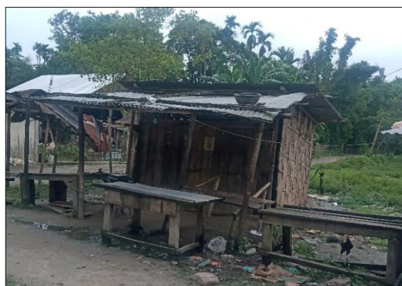
Exhibit-3: Temporary Structure
