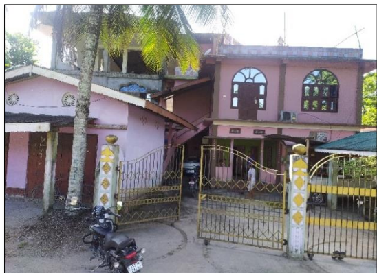
Exhibit-1: Permanent Structure
