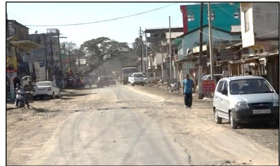
Exhibit-4: Road Condition
