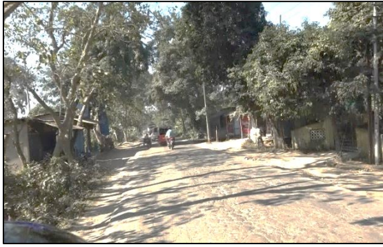
Exhibit-1: Road Condition
