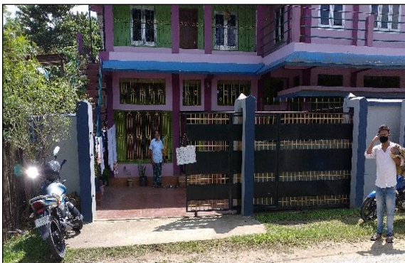
Exhibit-1: Permanent residential Structure
