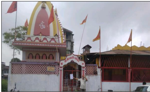
Exhibit-1: Temple along the project road
