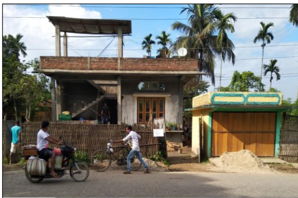
Exhibit-1: Permanent Structure
