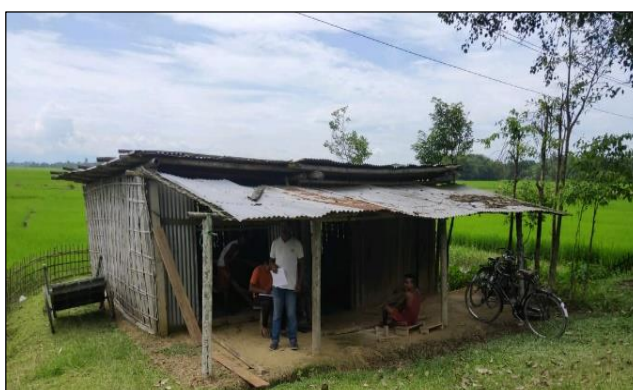
Exhibit-3: Temporary Structure
