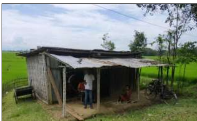
Exhibit-3: Temporary Structure
