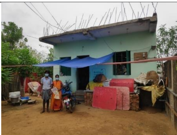
Asset No.AK-27 - Ammamambakkam Settlement
