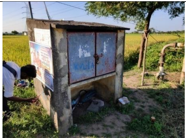
Asset No.KVL-1A Karikalavakkam Settlement
