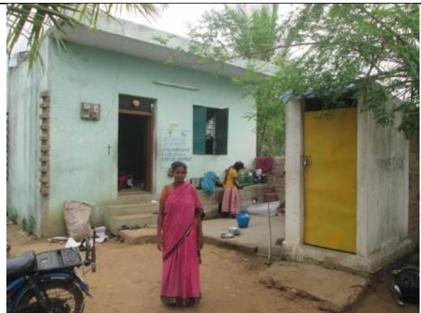
Asset No.AK-26 - Ammamambakkam Settlement
