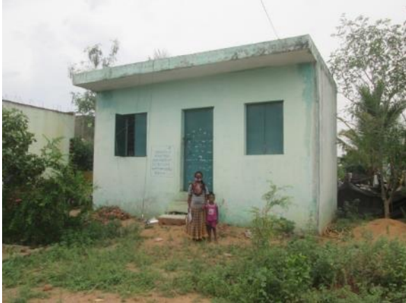
Asset No.AK-16 - Ammamambakkam Settlement
