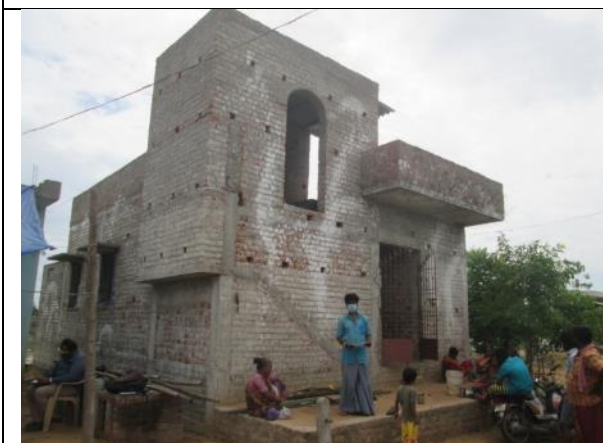
Asset No.AK-46 - Ammamambakkam Settlement
