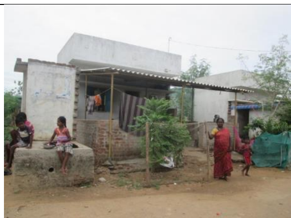
Asset No. AK-3 - Ammamambakkam Settlement
