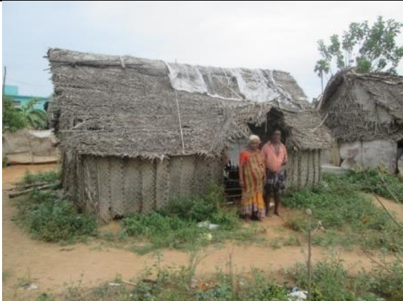
Asset No.AK-61 - Ammamambakkam Settlement
