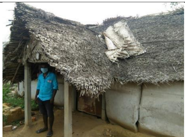
Asset No.AK-60 - Ammamambakkam Settlement
