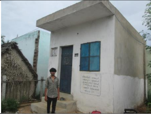
Asset No.AK-23 - Ammamambakkam Settlement
