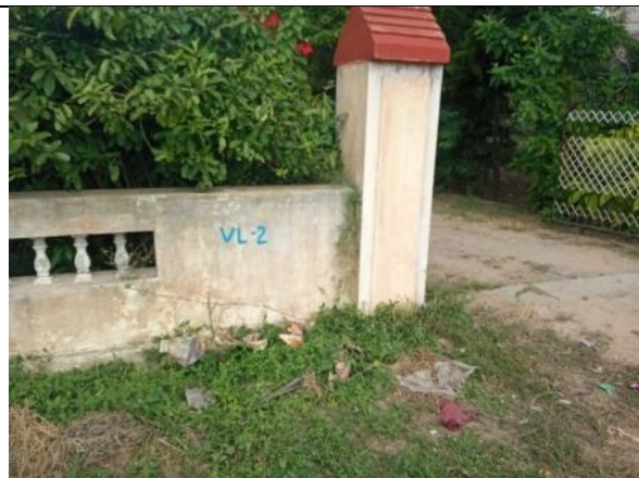
Asset No. VKL-2 - Vishnuvakkam Settlement
