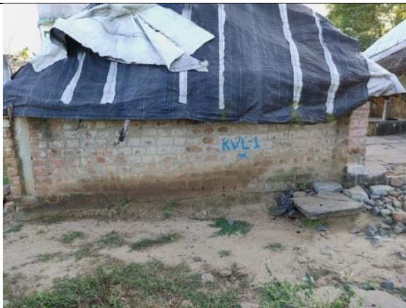
Asset No.KVL-1 Karikalavakkam Settlement
