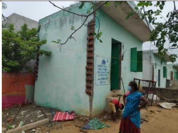
Asset No.AK-11 - Ammamambakkam Settlement
