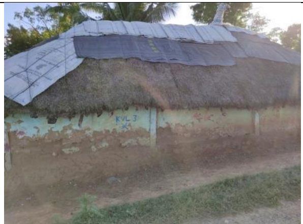
Asset No.KVL-3 Karikalavakkam Settlement
