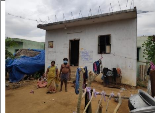
Asset No.AK-29 - Ammamambakkam Settlement
