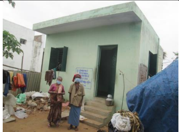
Asset No.AK-30 - Ammamambakkam Settlement
