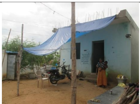
Asset No.AK-47 - Ammamambakkam Settlement
