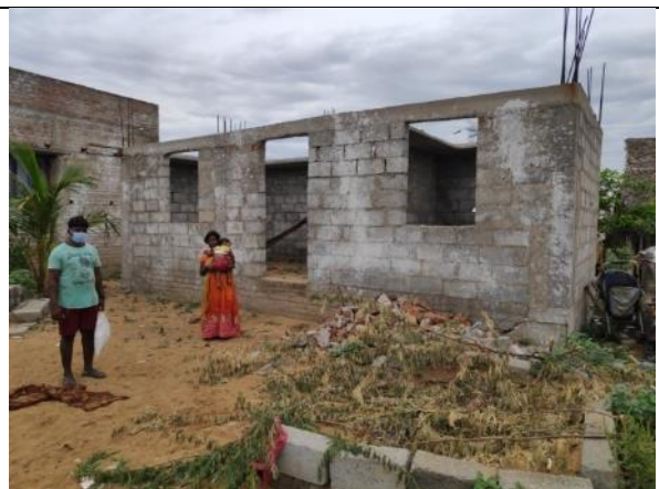
Asset No.AK-45 - Ammamambakkam Settlement
