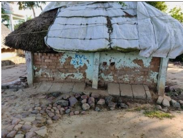
Asset No.KVL-2 Karikalavakkam Settlement
