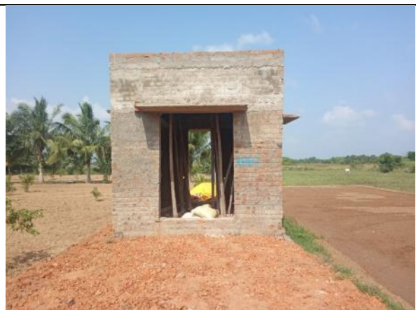
Asset No. KPR-1 - Kilampakkam Settlement
