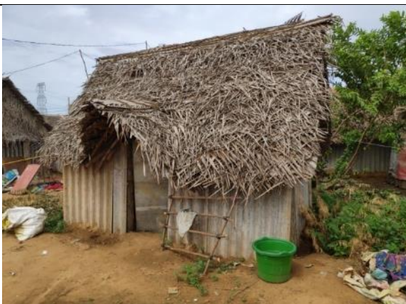
Asset No.AK-65 - Ammamambakkam Settlement
