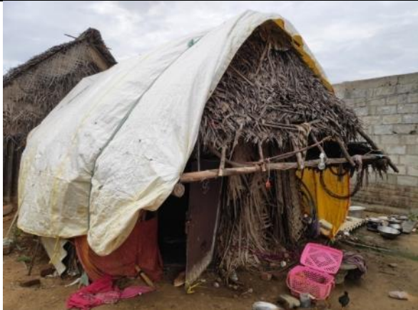
Asset No.AK-48 - Ammamambakkam Settlement
