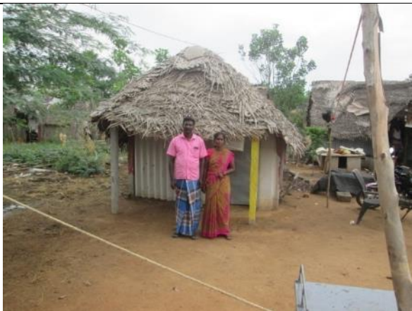
Asset No.AK-57 - Ammamambakkam Settlement
