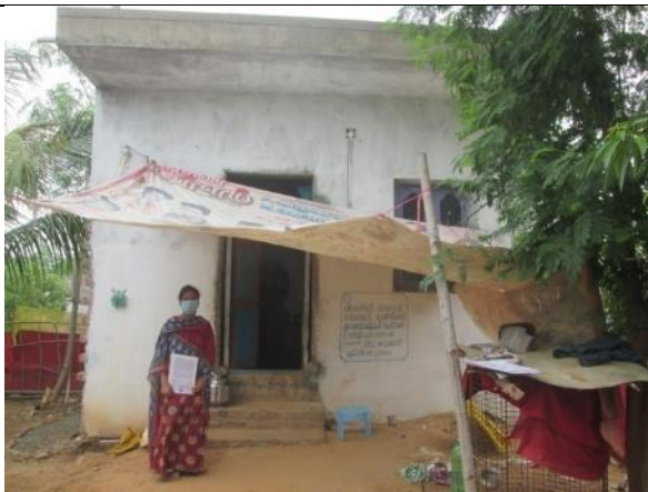
Asset No.AK-25 - Ammamambakkam Settlement
