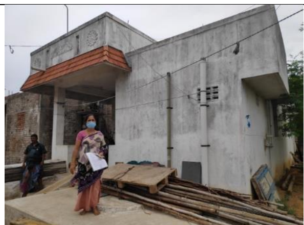
Asset No.AK-34 - Ammamambakkam Settlement
