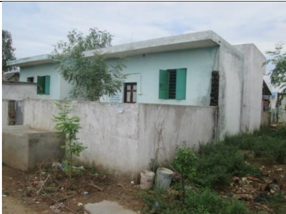
Asset No.AK-10 - Ammamambakkam Settlement
