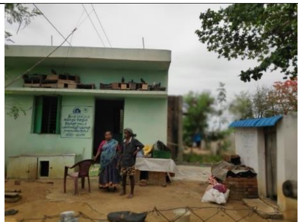
Asset No.AK-28 - Ammamambakkam Settlement
