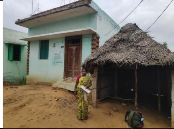
Asset No.AK-24 - Ammamambakkam Settlement
