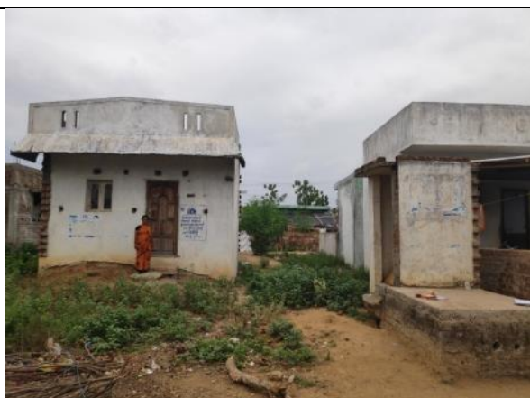
Asset No. AK-2 - Ammamambakkam Settlement
