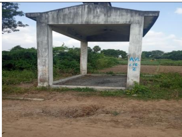
Asset No. AVL-2 Athivakkam Village
