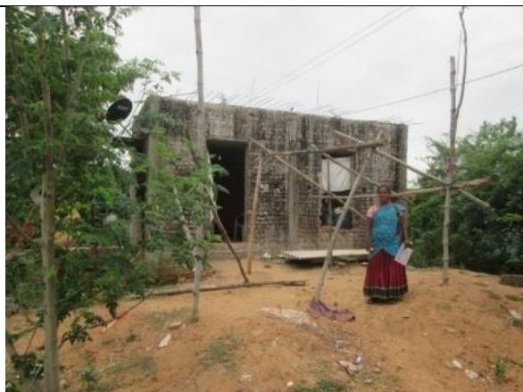
Asset No.AK-39 - Ammamambakkam Settlement
