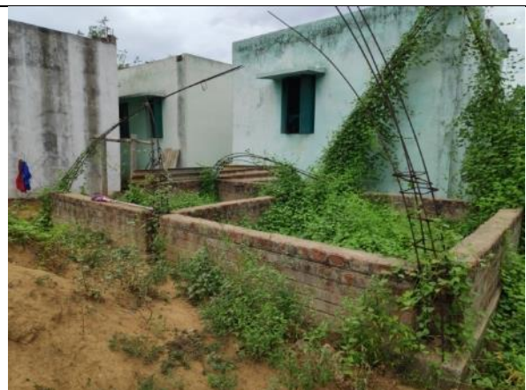
Asset No.AK-32 - Ammamambakkam Settlement
