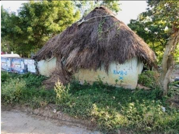
Asset No.KVR-1 - Karikalavakkam Settlement
