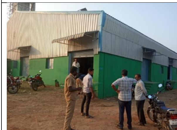
Asset No. PPR-1 - Punnappakkam Settlement
