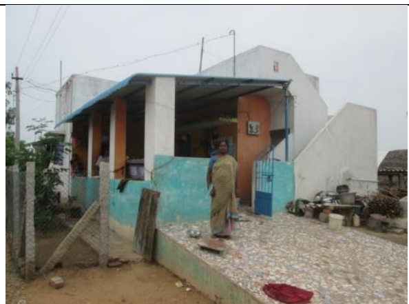
Asset No.AK-7 - Ammamambakkam Settlement
