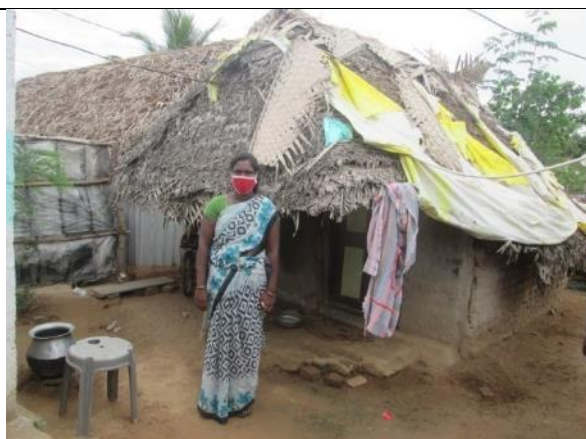
Asset No.AK-54 - Ammamambakkam Settlement
