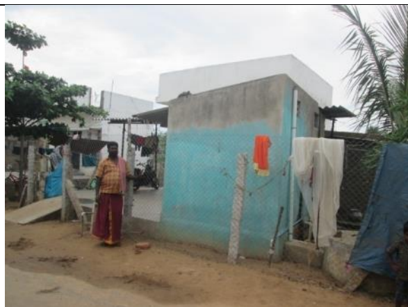
Asset No.AK-6 - Ammamambakkam Settlement
