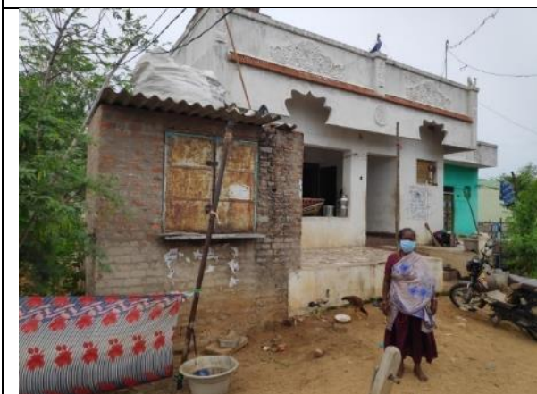
Asset No.AK-33 - Ammamambakkam Settlement
