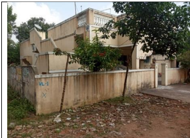
Asset No. VKL -1 - Vishnuvakkam Settlement
