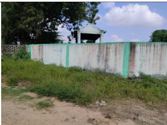
Asset No. AVL-1 Athivakkam Village
