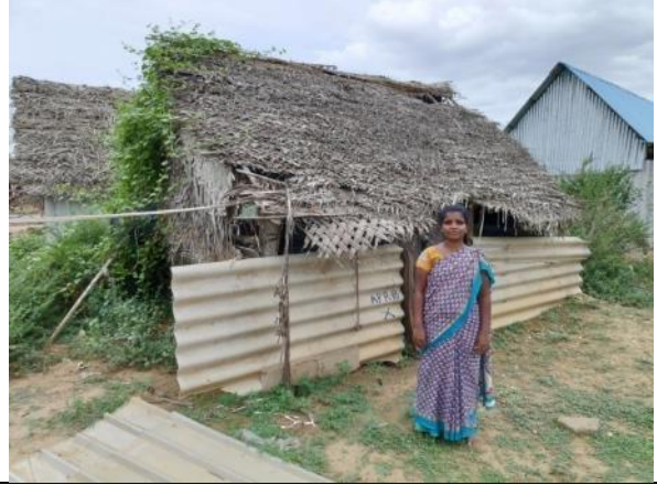
Asset No.AK-68 - Ammamambakkam Settlement
