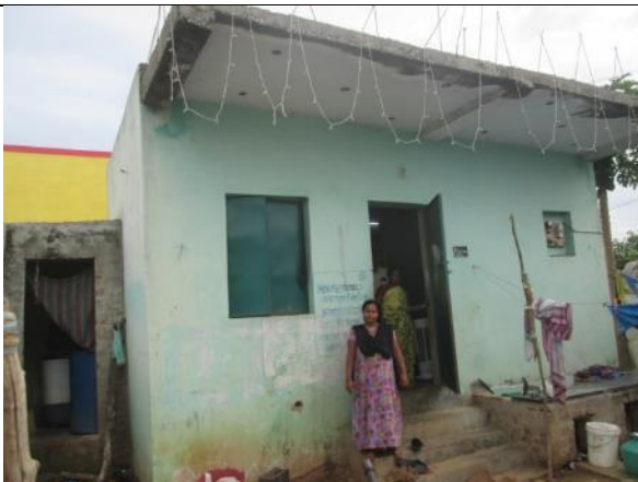
Asset No.AK-21 - Ammamambakkam Settlement
