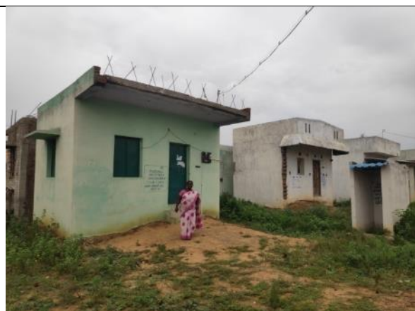
Asset No. AK-1 - Ammamambakkam Settlement
