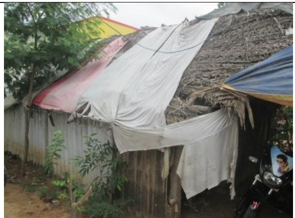
Asset No.AK-22 - Ammamambakkam Settlement
