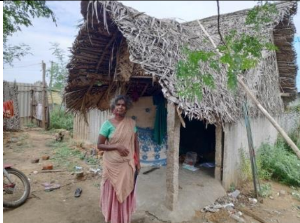
Asset No.AK-49 - Ammamambakkam Settlement
