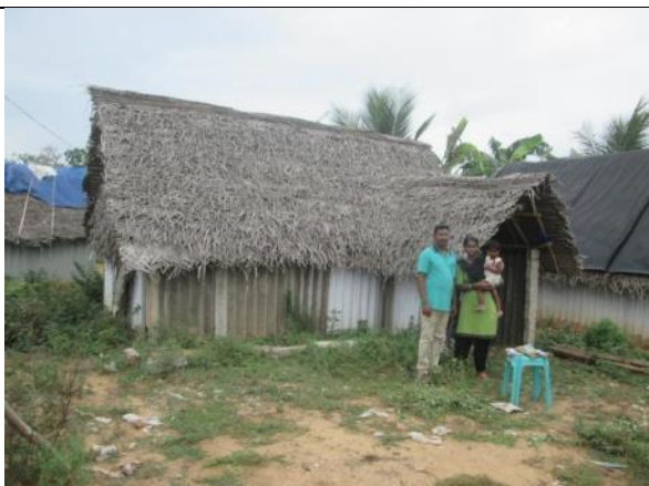
Asset No.AK-51 - Ammamambakkam Settlement
