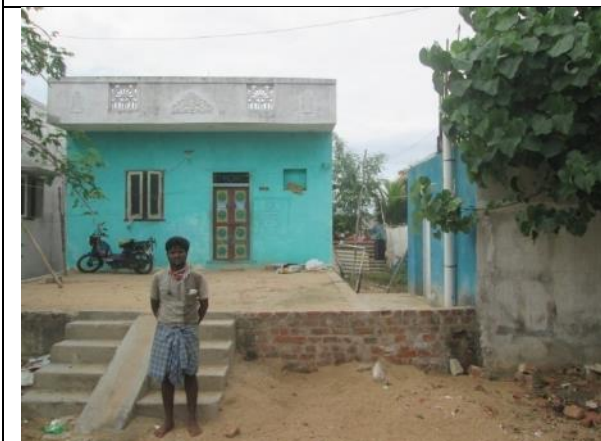
Asset No.AK-31 - Ammamambakkam Settlement
