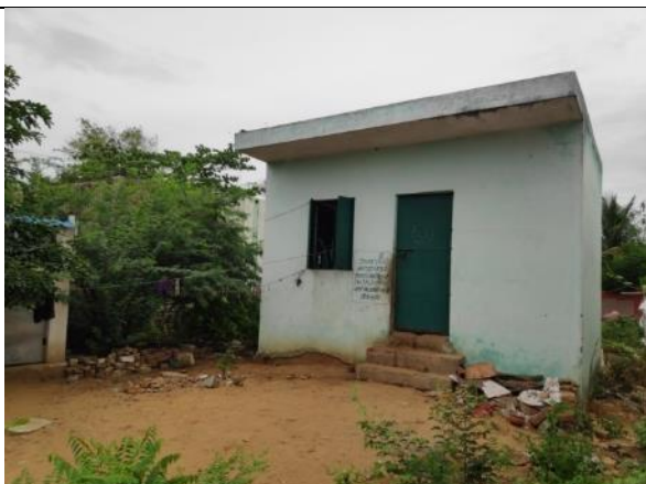
Asset No.AK-38 - Ammamambakkam Settlement
