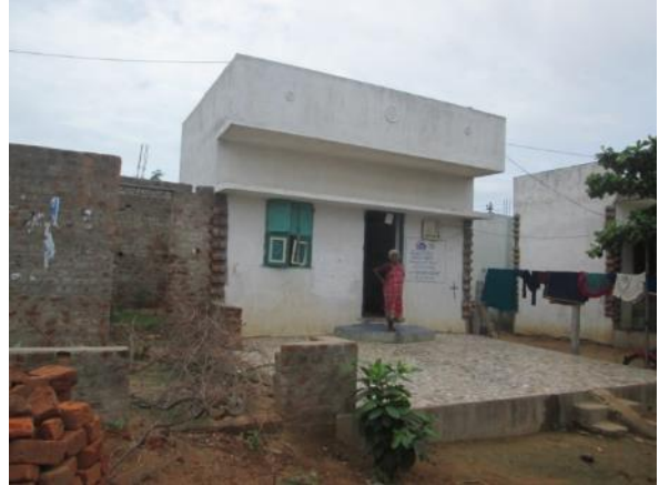
Asset No.AK-5 - Ammamambakkam Settlement
