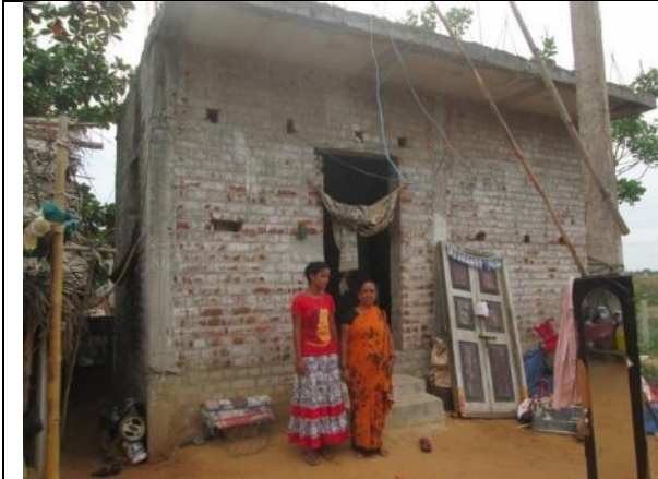
Asset No.AK-42 - Ammamambakkam Settlement
