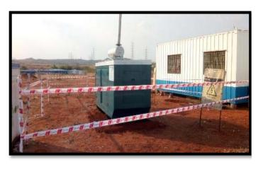
Figure 2.5 62.5 kV DG set at Site
