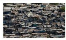
Our data suggest that the project is located in a region where Peak Ground Acceleration (PGA) of >31 cm/s may be expected from a 250j return period event, potentially leading to moderate to heavy damage. This is based on postprocessed data from International Centre for Numerical Methods in Engineering (CIMNE) and INGENIAR Ltda (GAR15).
