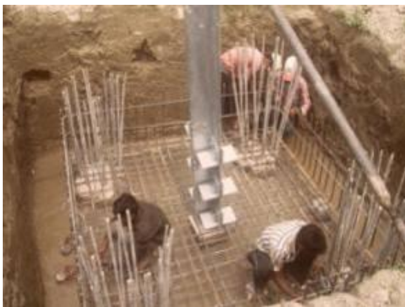
Figure 3.15: Striping the tower footing with steel
