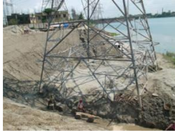
Figure 3.18: Placing tower on its foundation
