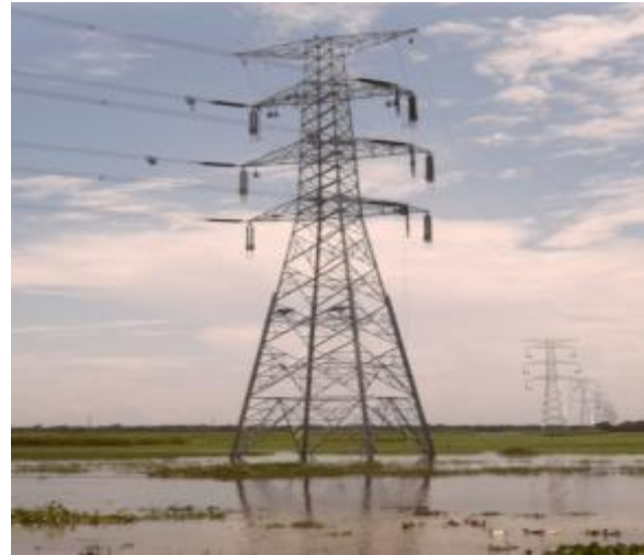
Figure 3.6: Suspension Tower
