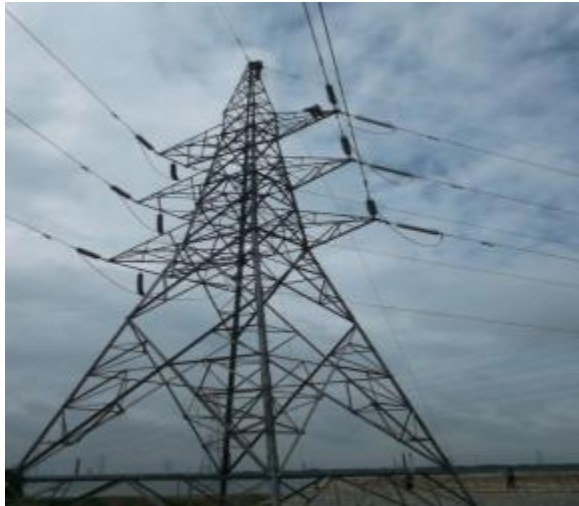
Figure 3.5: Angle Tower (Tension Tower)
