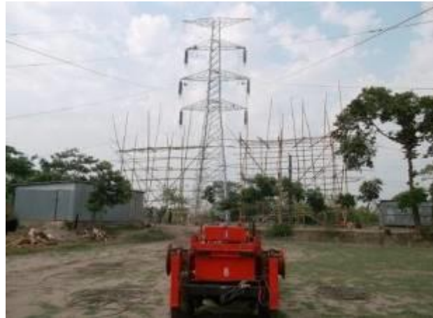
Figure 3.20: Conductor stringing
