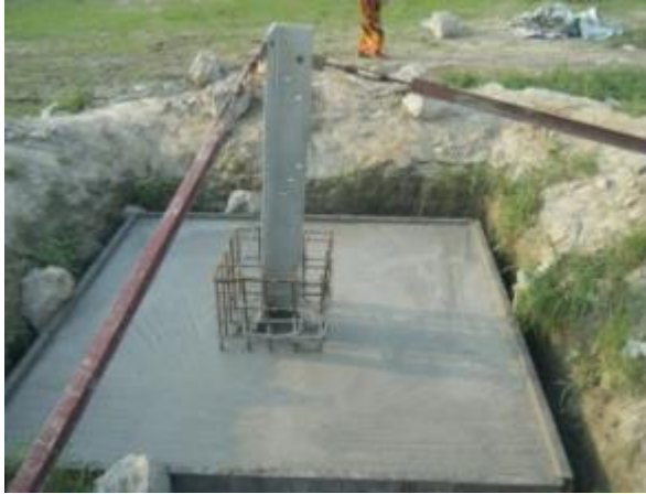
Figure 3.17: Casting concrete cement into tower foundation
