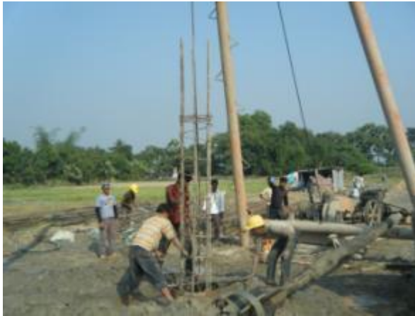
Figure 3.11: Placing steel ring bunds
