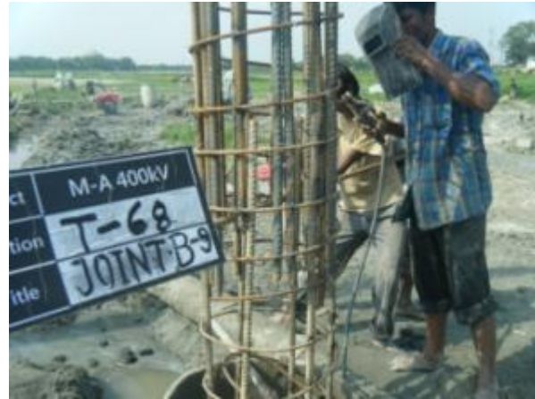
Figure 3.12: Welding of reinforcements
