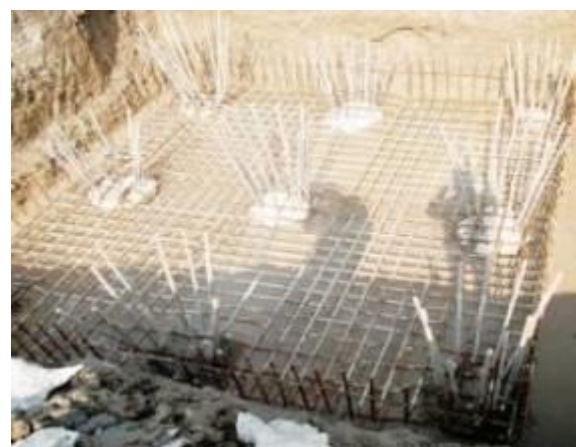
Figure 3.14: Pile cap reinforcement
