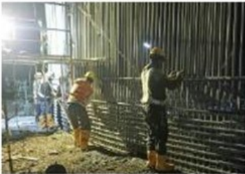
Wall Rebar Installation
