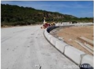
Kerb Barrier at Roundabout P2
