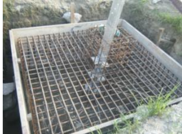
Figure 3.16: Providing detail reinforcements
