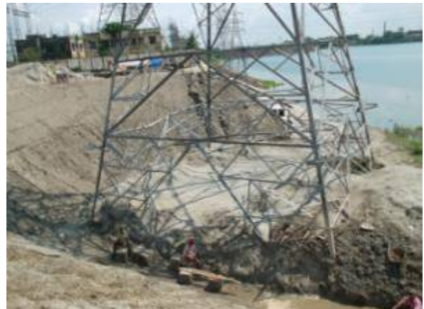
Figure 3.18: Placing tower on its foundation
