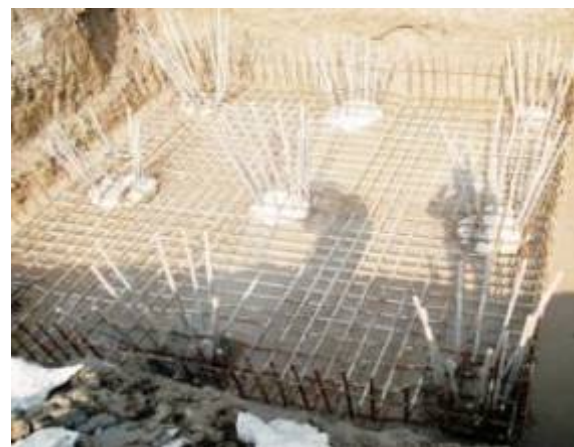
Figure 3.14: Pile cap reinforcement
