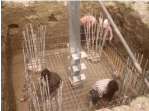
Figure 3.15: Striping the tower footing with steel
