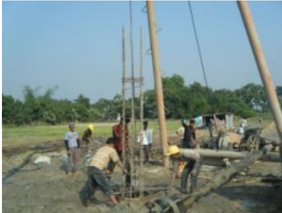
Figure 3.11: Placing steel ring bunds
