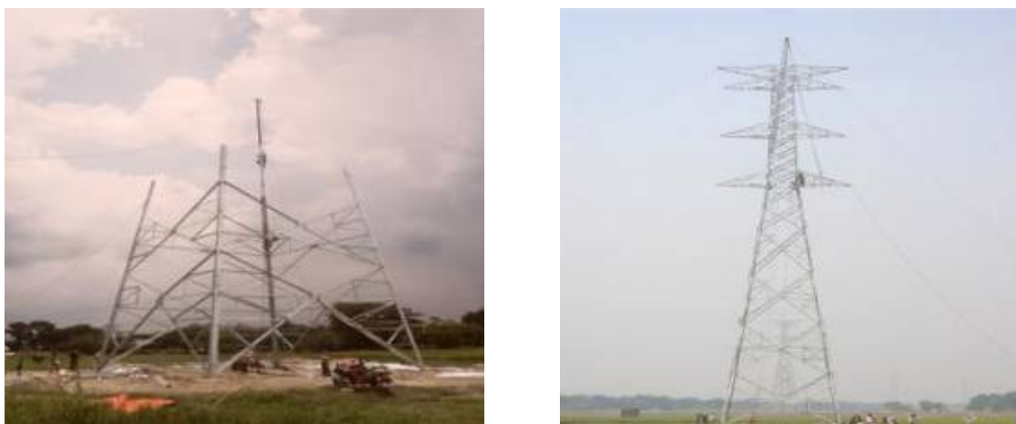
Figure 3.19: Tower erection works
