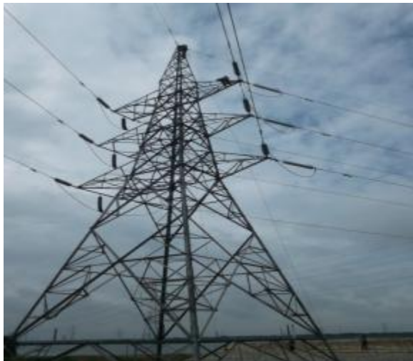
Figure 3.5: Angle Tower (Tension Tower)
