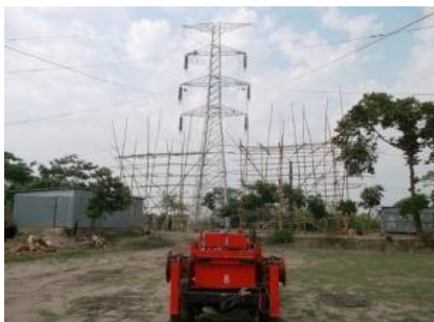
Figure 3.20: Conductor stringing
