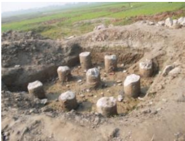
Figure 3.13: Tower piling work
