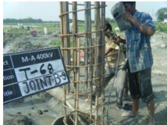
Figure 3.12: Welding of reinforcements
