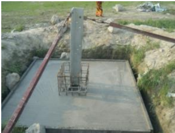
Figure 3.17: Casting concrete cement into tower foundation
