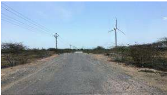
Present bituminous surface deteriorated since surface is more than 7 years old.
