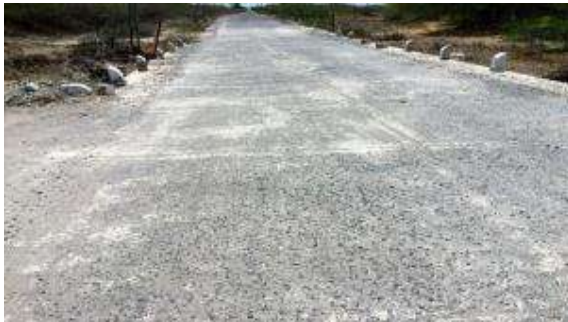
Cement concrete surface of culvert is deteriorated since surface is more than 7 years old.
