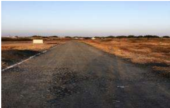
Road Construction Work Under Progress; Bituminous yet to lay
