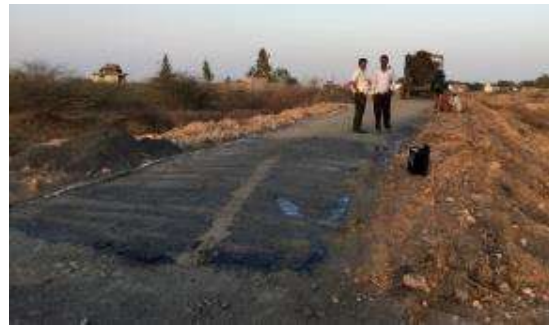
Bituminous laying under progress
