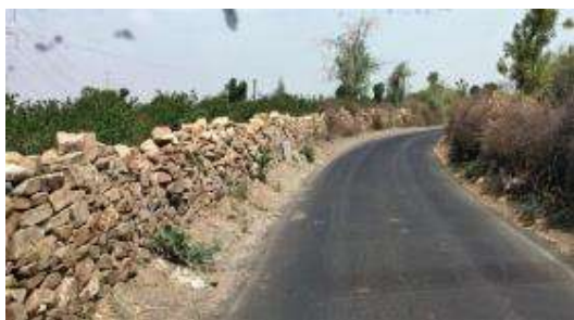
Encroachment of shoulder and side drain upto carriageway
