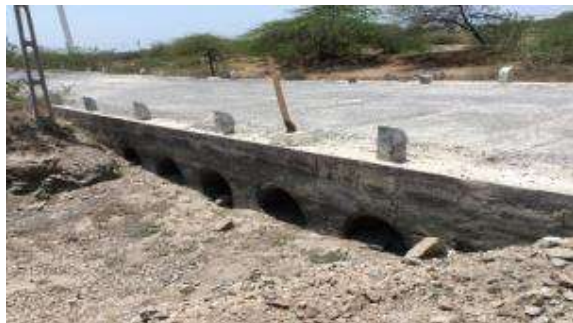
Existing level of Culvert is low and problem of water overtopping prevails in rainy season.
