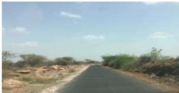
One BT Layer has just been laid providing smooth riding quality to the commuters
